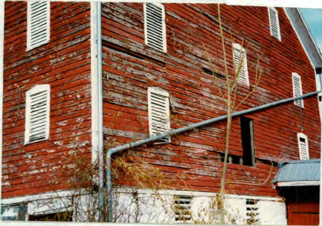
Detail of work needed on Barn,
