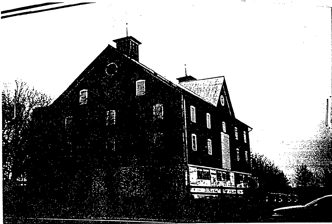
Barn viewed from street
