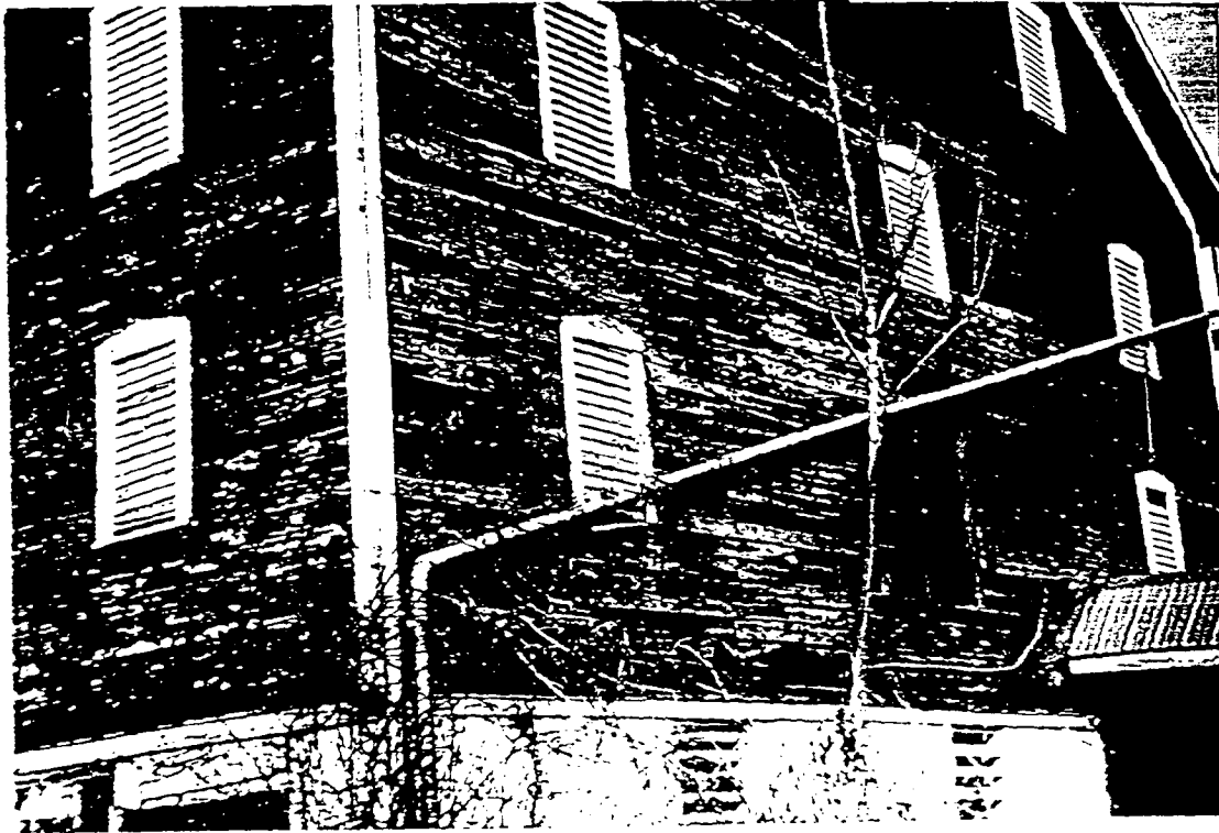
Detail of work needed on Barn.
