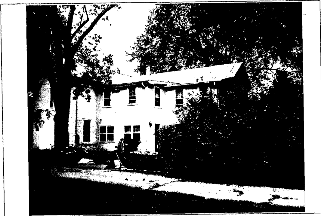
Detail: Roof - Notice Flat Roof Areas
