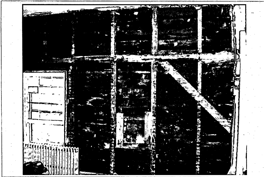
Detail: Extensive Termite Damage on Eastern Wall Due to leaking Roof. (Bedroom)
