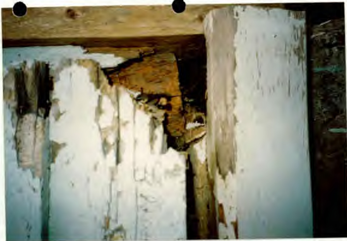
Termite.. Damage
