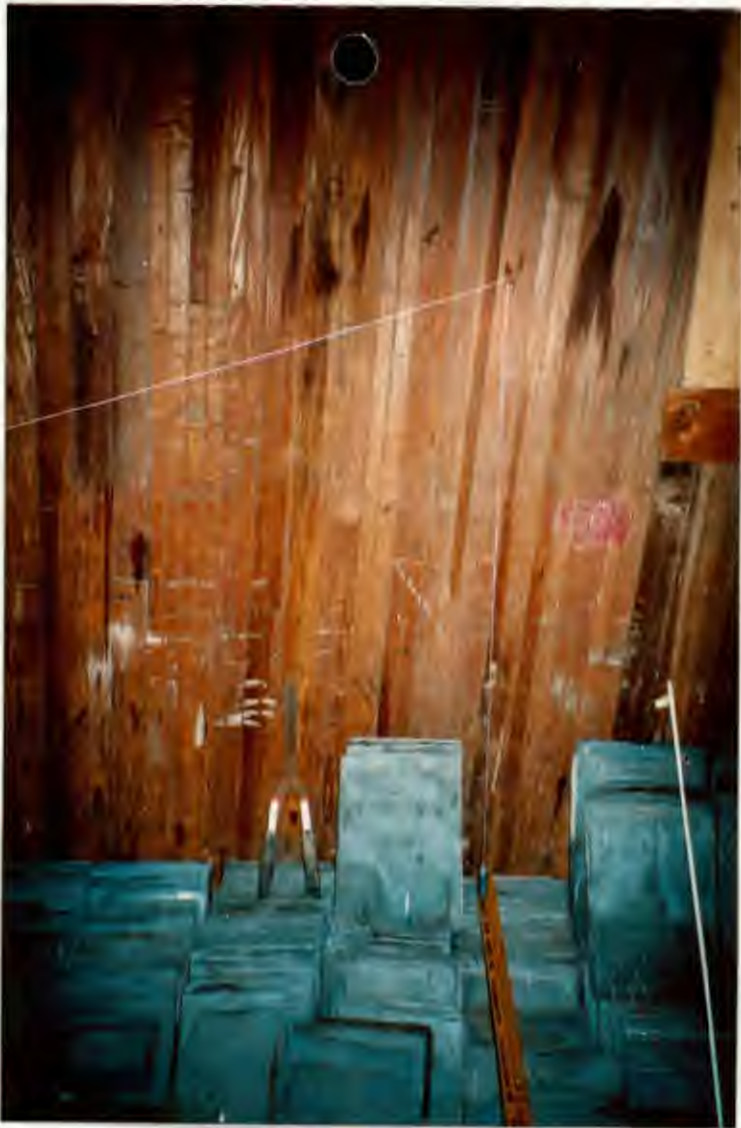
Back Wall with Plumb Line
