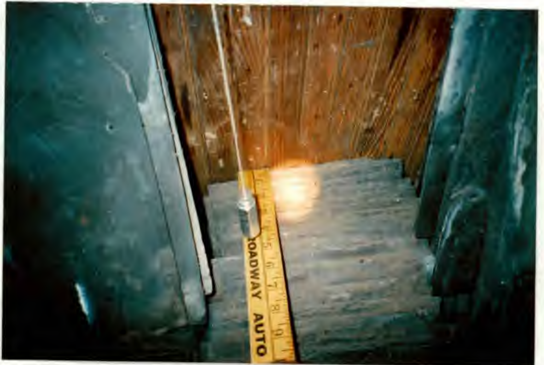
Back Wall with Plumb Line
