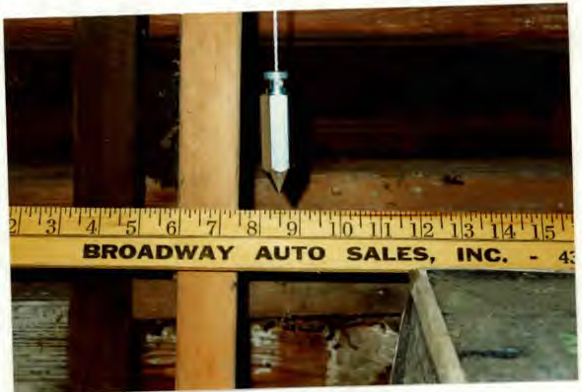
Right Wall with Plumb Line
