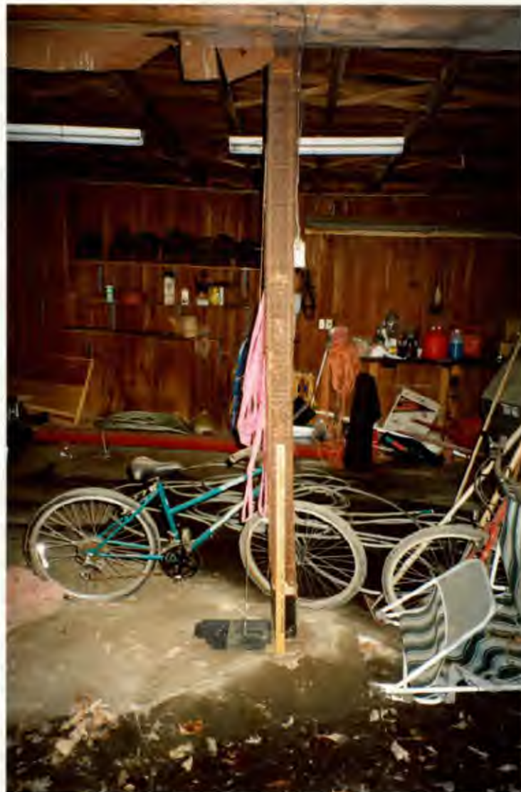
A Center Column with Plumb Line
