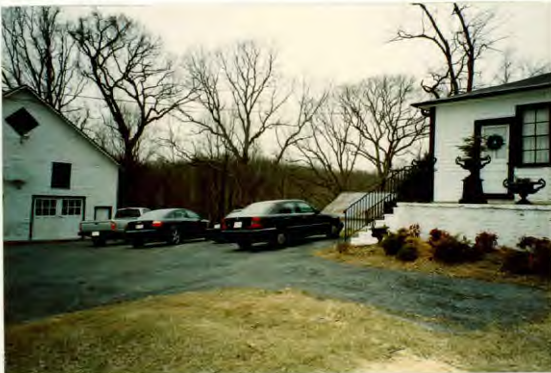
SHED VIEWED FROM FRONT OF HOUSE
