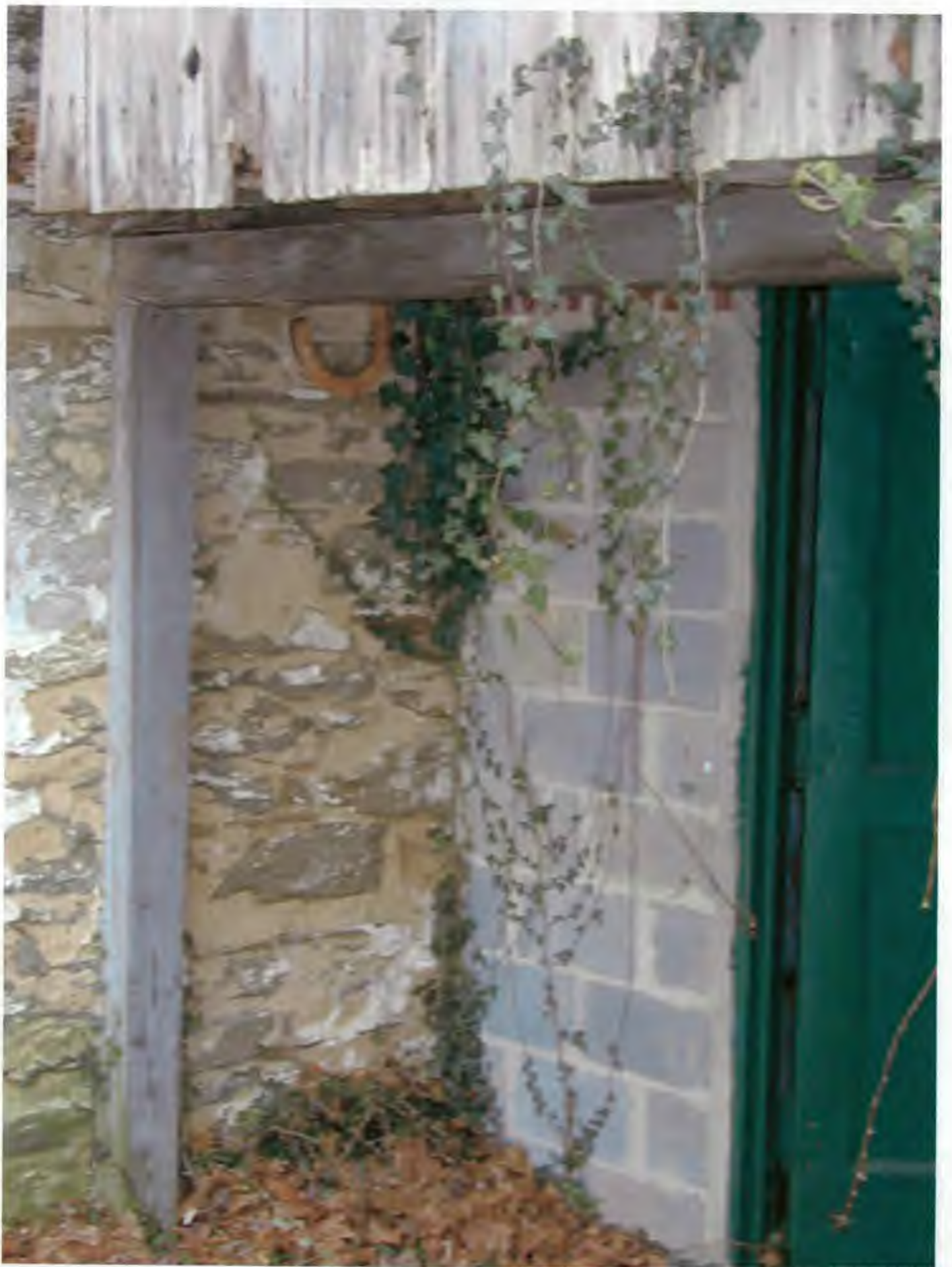
WOODLAWN HISTORIC STONE BARN NORTH ELEVATION (EXISTING POST)
