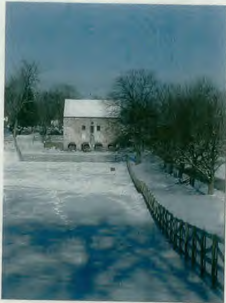
WOODLAWN HISTORIC STONE BARN (FROM EDNOR RD)
