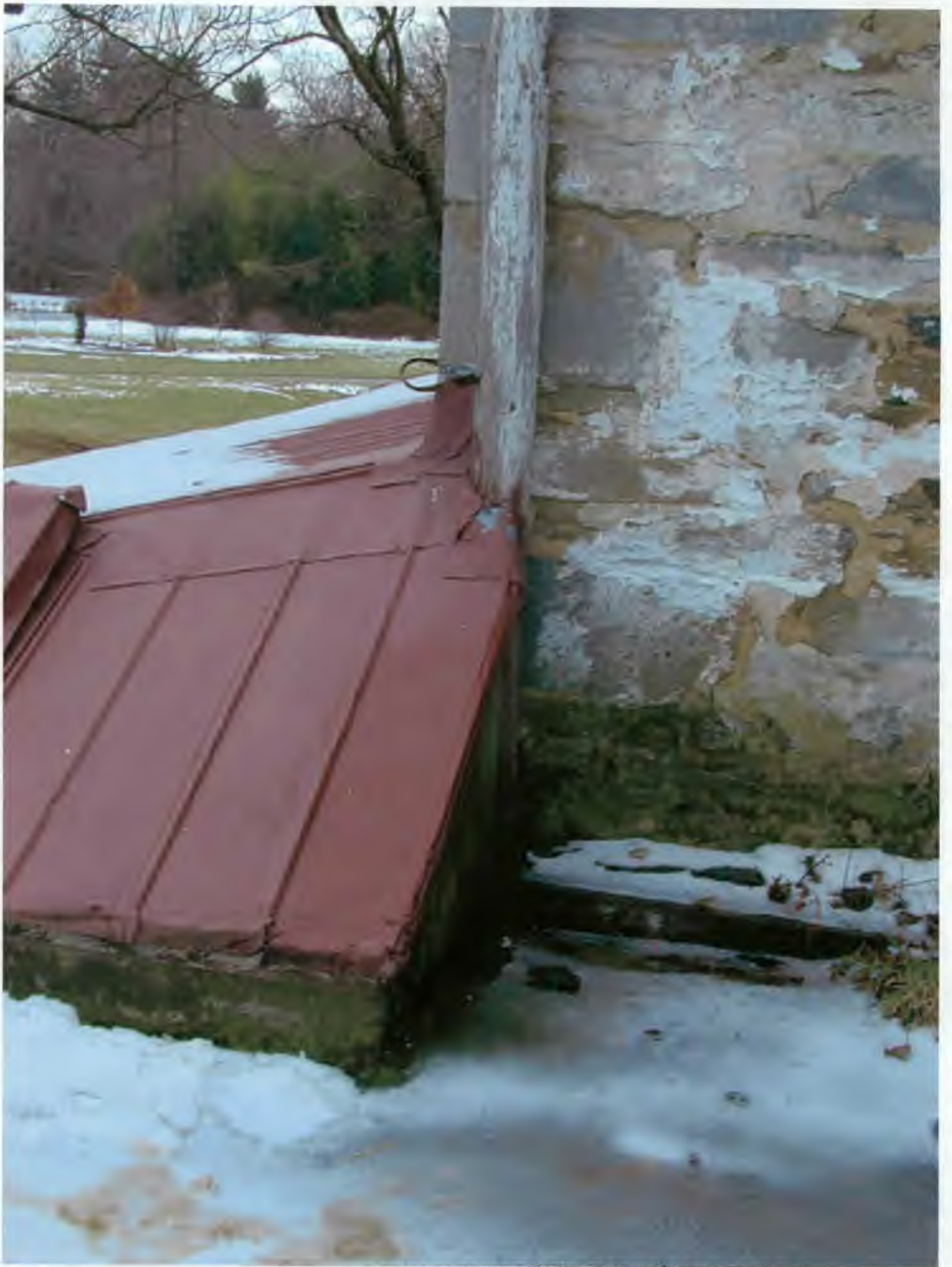
WOODLAWN HISTORIC STONE BARN NORTH ELEVATION (EXISTING SHED ROOF)
