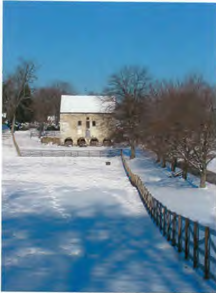
WOODBLOWN HISTORIC STONE BARN (FROM EDNOR RD)
