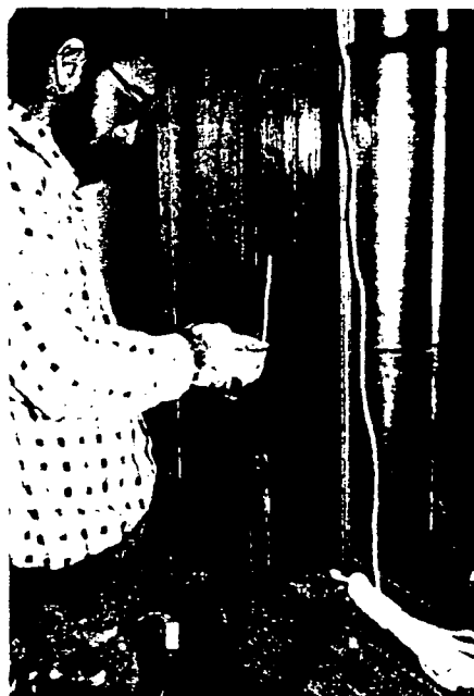
Figure 4e. A common repair is the replacement of broken sash cords with new cords (shown) or with chains. The weight pocket is often accessible through a removable plate in the jamb, or by removing the interior trim. Photo: John H. Myers
