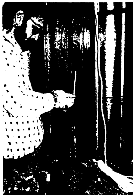
Figure 4e. A common repair is the replacement of broken sash cords with new cords (shown) or with chains. The weight pocket is often accessible through a removable plate in the jamb, or by removing the interior trim. Photo: John H. Myers
