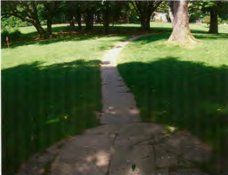
Detail: View of existing walkway leading from hemlock grove to mansion.
