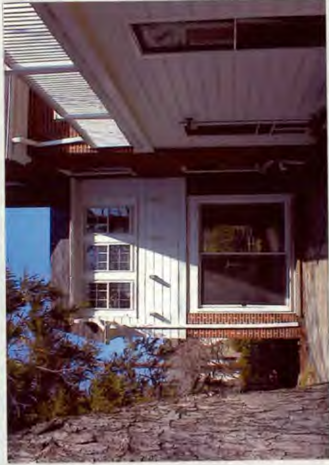
⑥ VIEW OF EXISTING SIDE ADDITION - REAR FAÇADE
