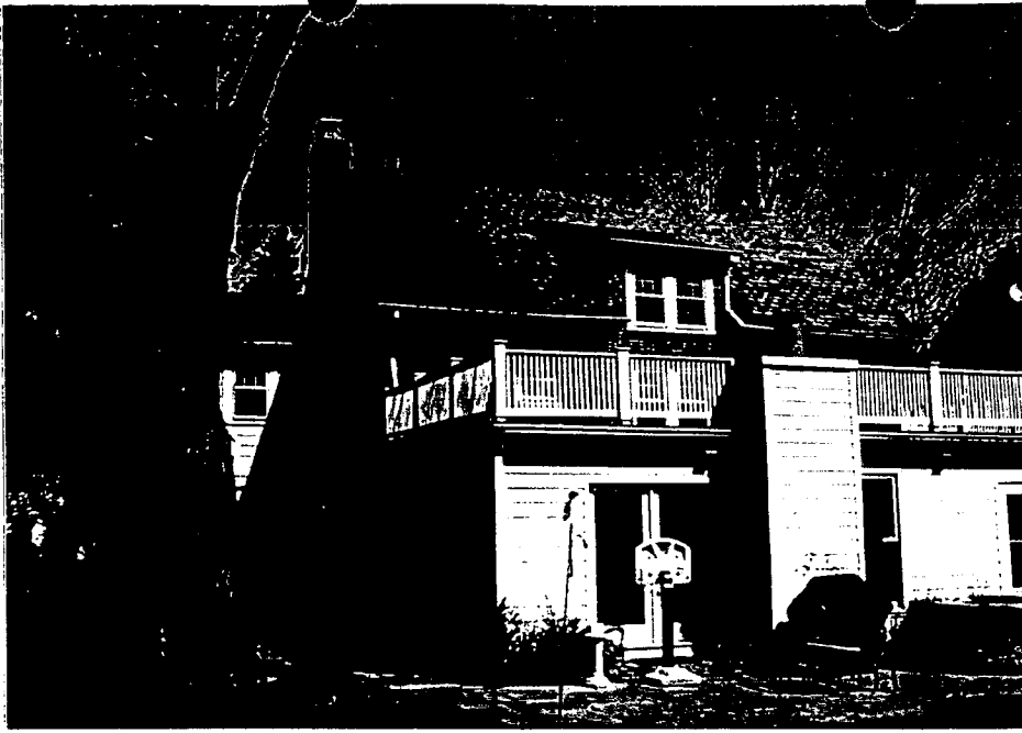
⑦ VIEW OF REAR FACADE, WITH THE RECENT FLAT-ROOF ADDITION.
