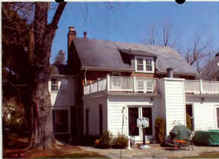
⑦ VIEW OF REAR FACADE, WITH THE RECENT FLAT-ROOF ADDITION.
