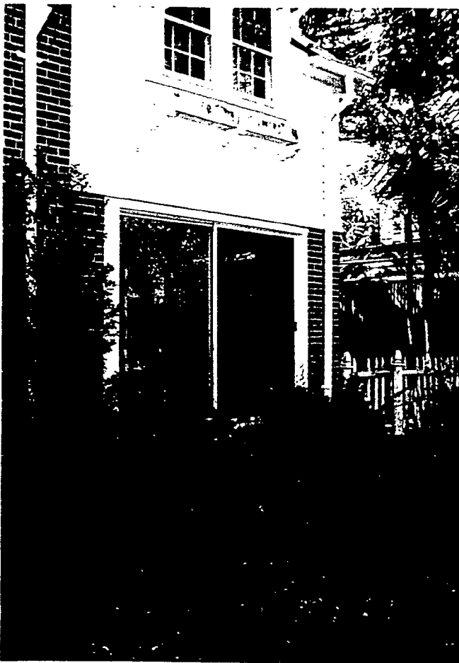
⑩B CLOSE-UP OF FRONT OF SUNROOM. THE EXISTING LANDSCAPING CONCEALS THE BOTTOM OF THE STRUCTURE.
