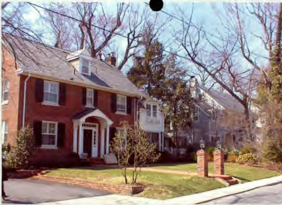
① VIEW OF THE HOUSE LOOKING WEST. PHOTO TAKEN FROM MIDDLE OF THE STREET
