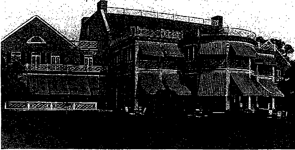
The west elevation of the Clubhouse after the addition of the semicircular bay.
