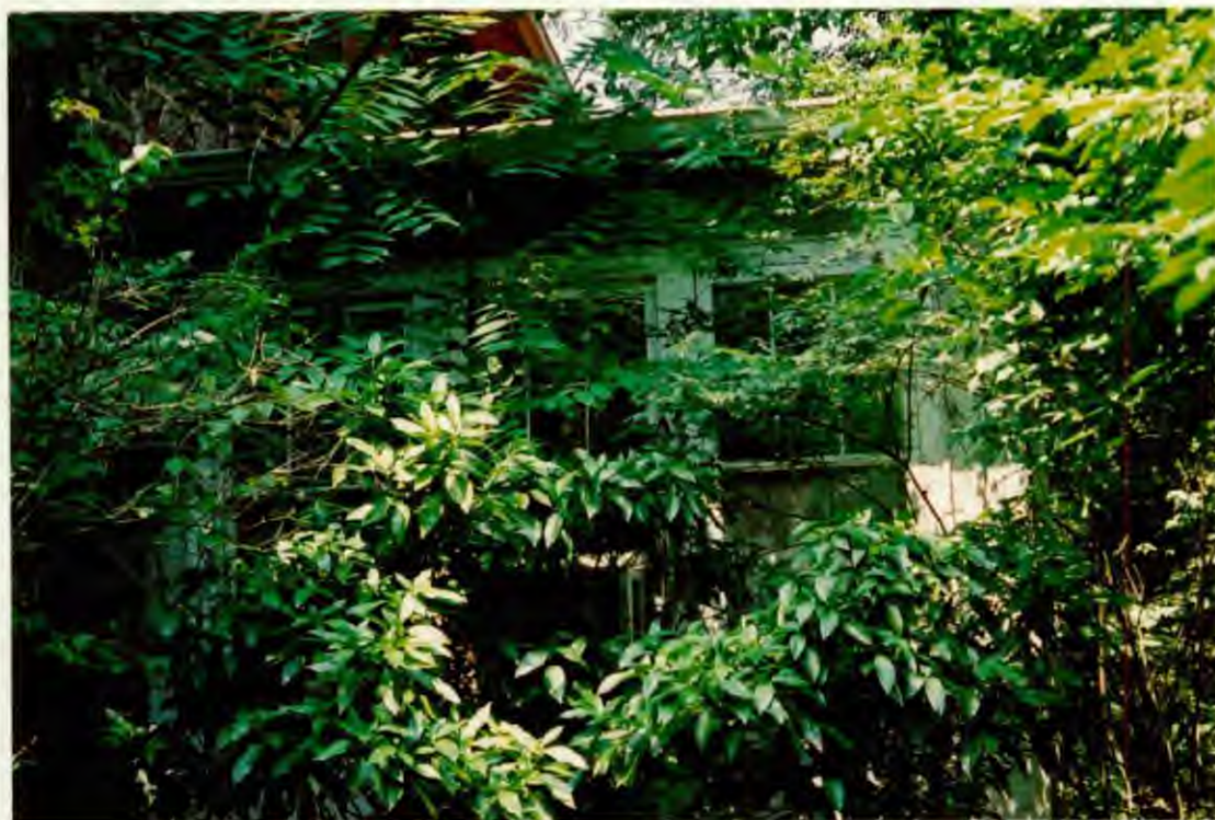
EAST SIDE - SOUTH WALL
