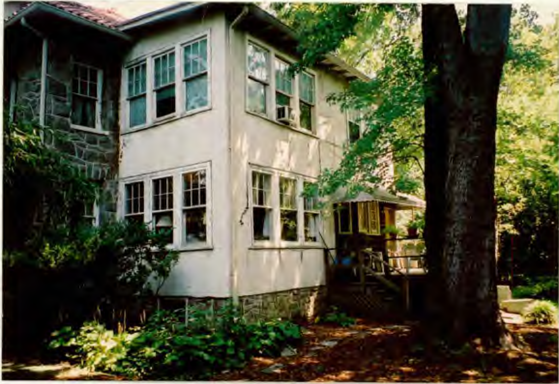
BACK - SW CORNER
