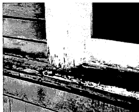
Deterioration of poorly maintained windows usually begins on horizontal surfaces and at joints, where water can collect and saturate the wood. Photo: NPS files.
