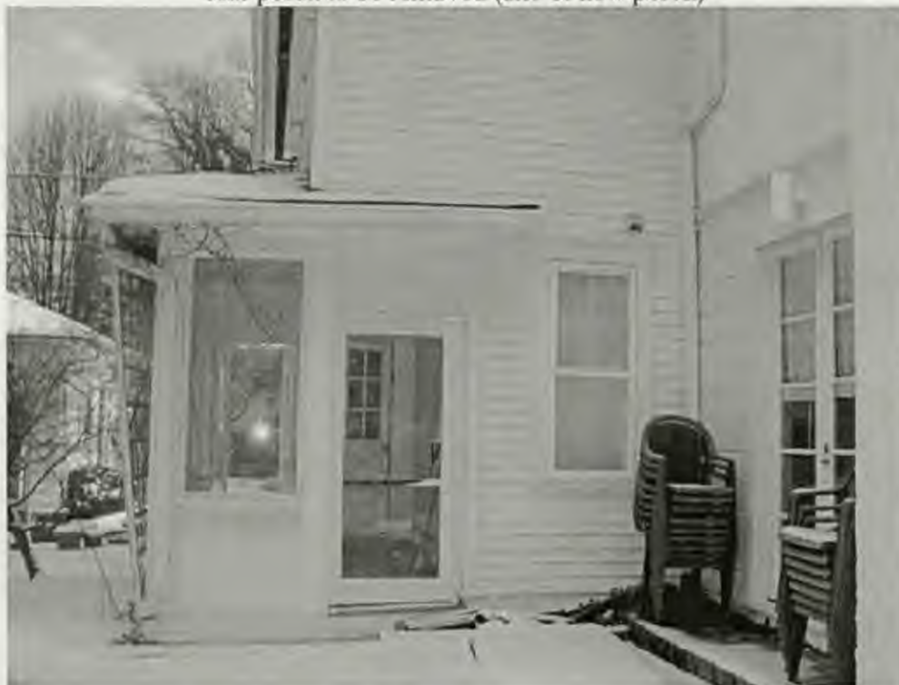
rear porch to be removed (site of new porch)
