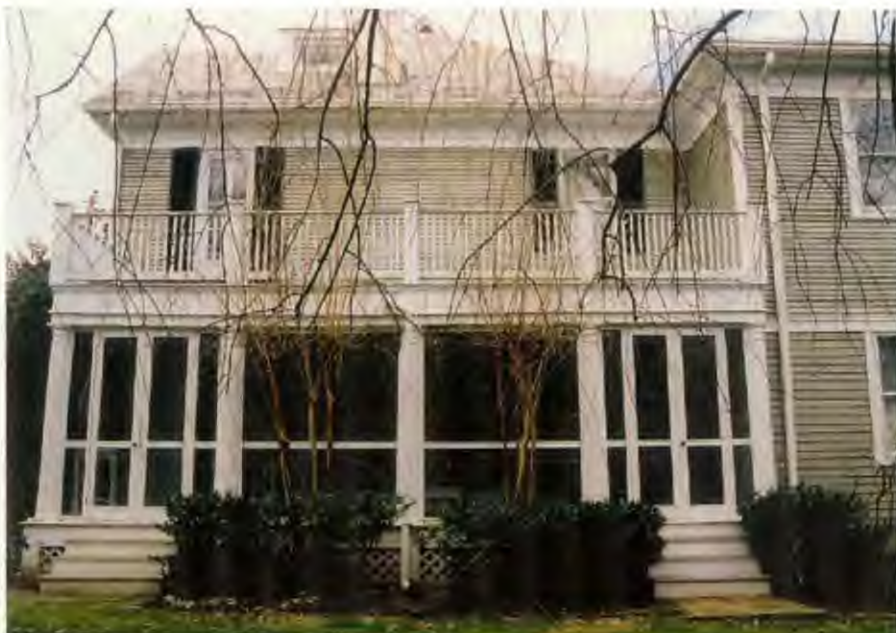
Existing East Elevation from sideyard.
