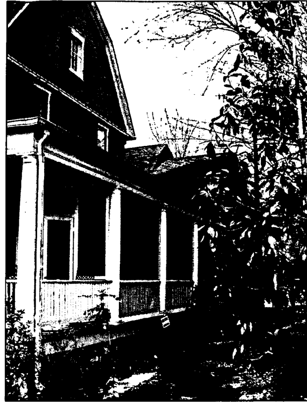
③ Existing Screened Porch No Scale
