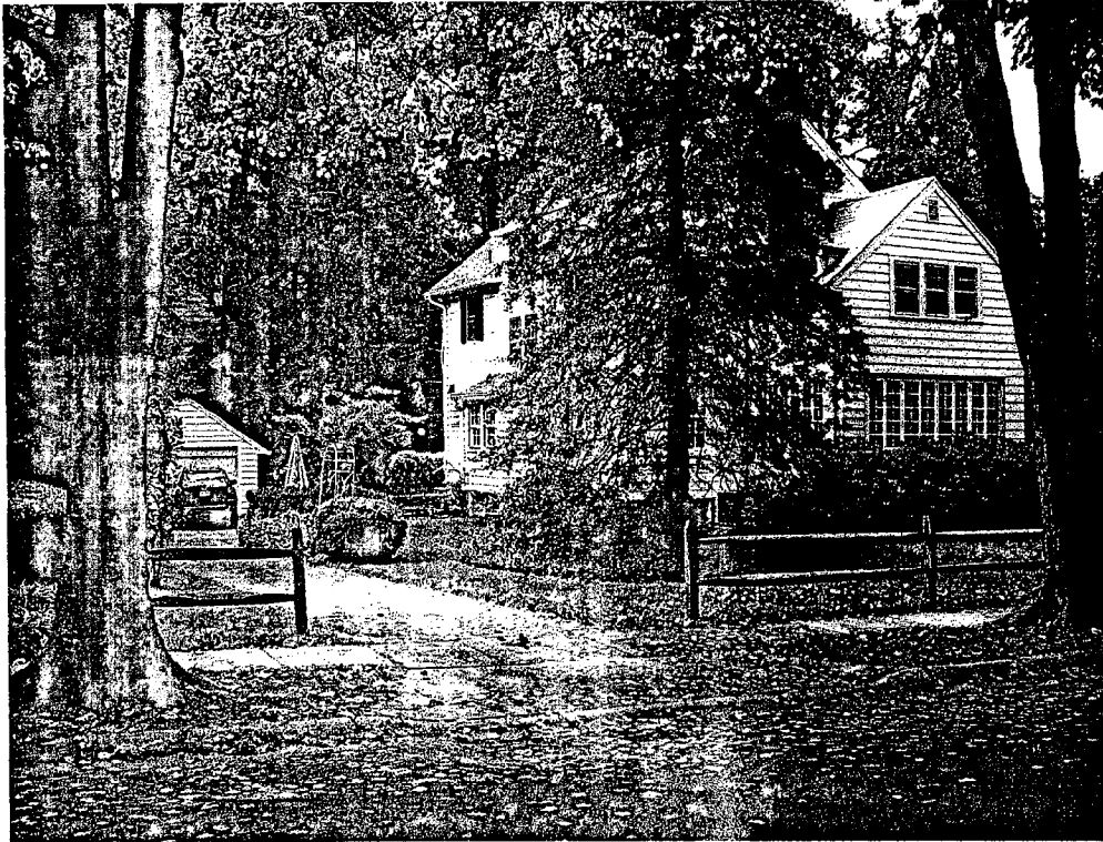
Driveway onto West Irving
