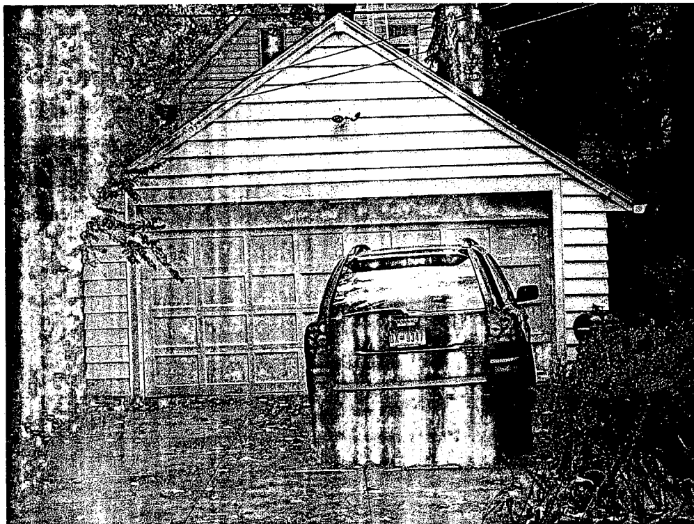
Existing garage from north
