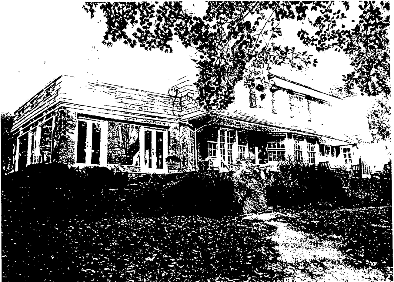
Rear (southwest) elevation from yard
