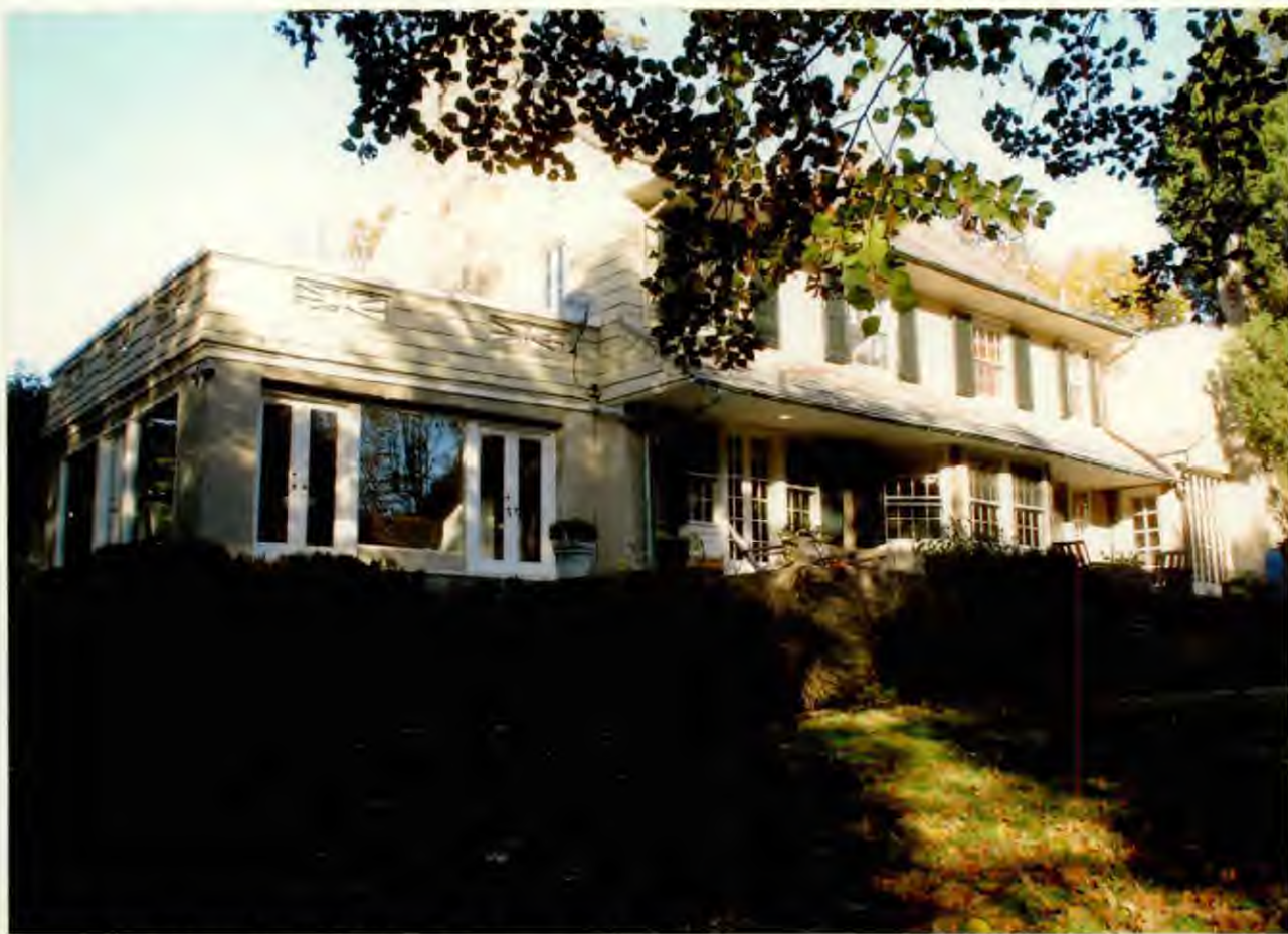
Rear (southwest) elevation from yard
