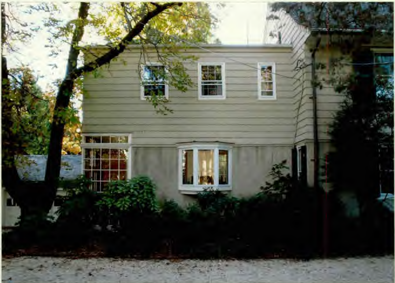
Detail, north elevation of existing addition
