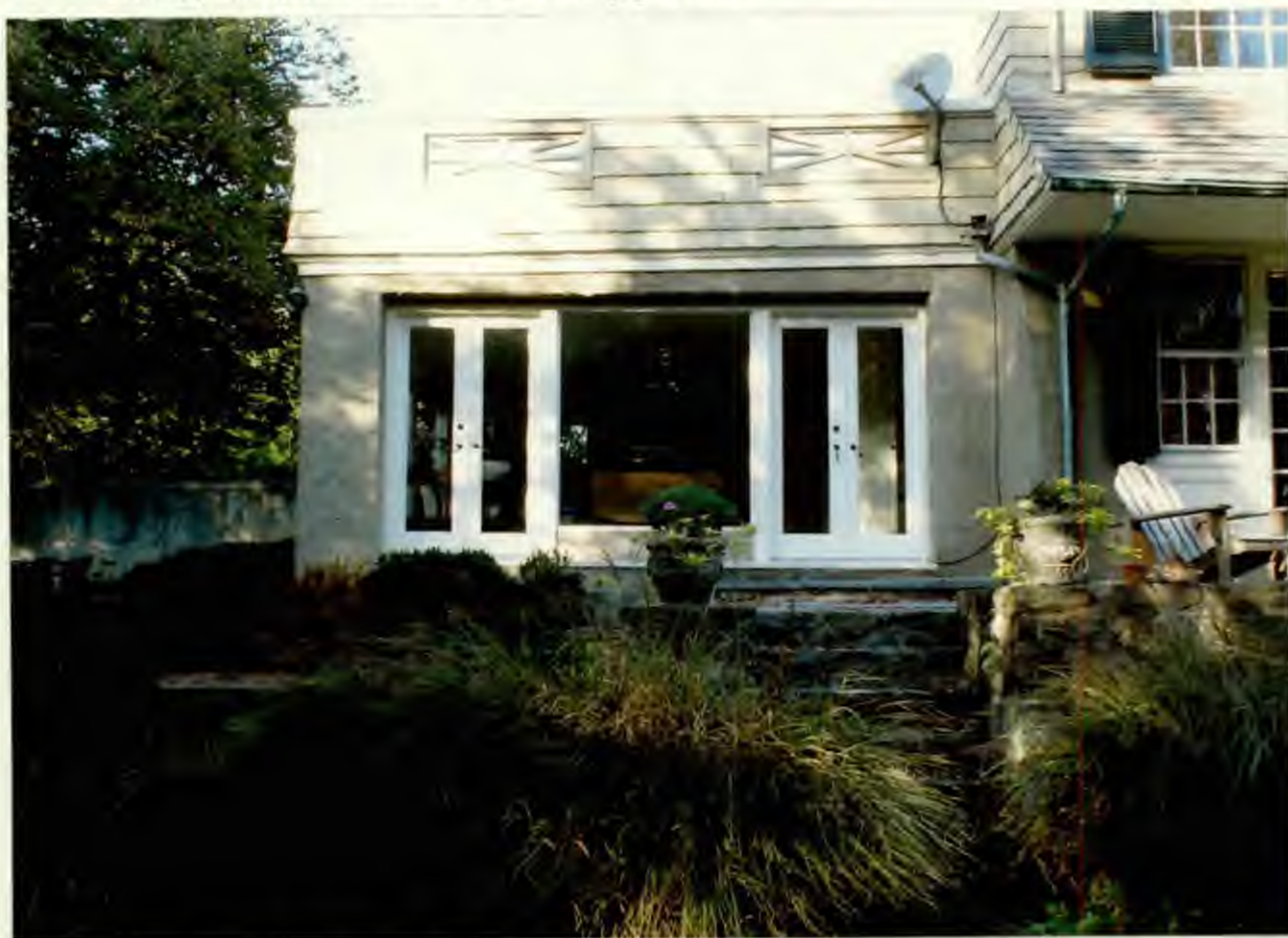
Detail, south elevation of existing one-story portion
