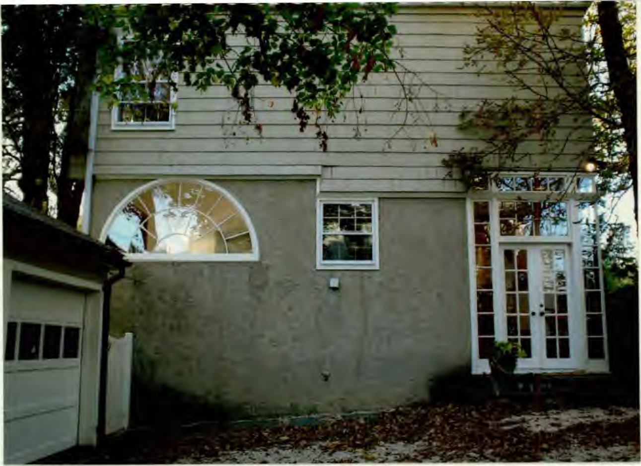
Detail, east elevation of existing addition
