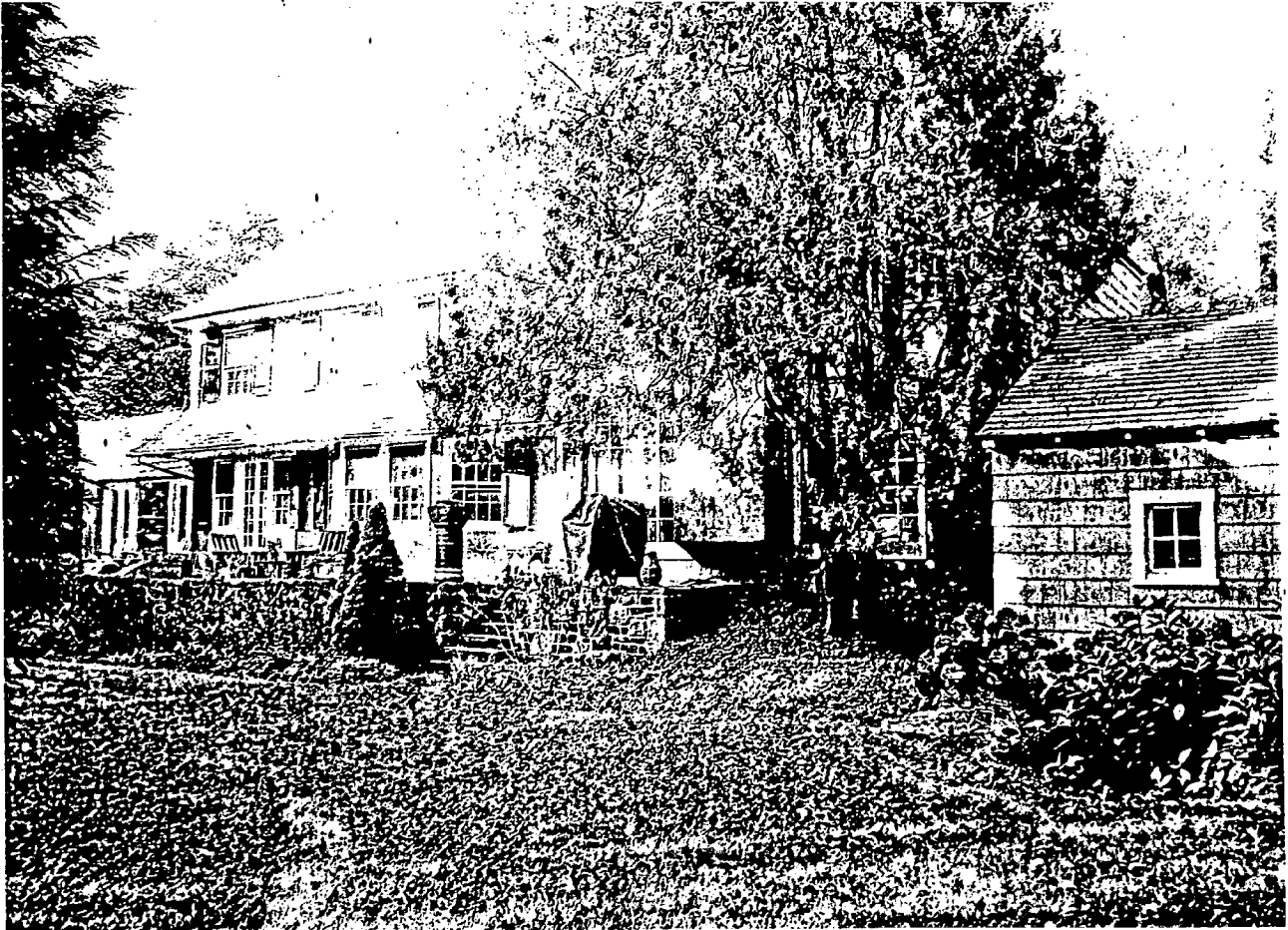
Rear (southeast) elevation from yard
