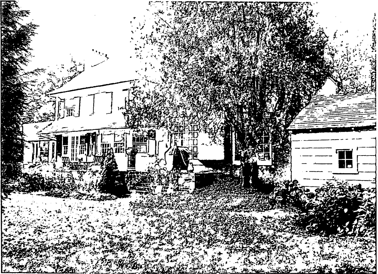
Rear (southeast) elevation from yard
