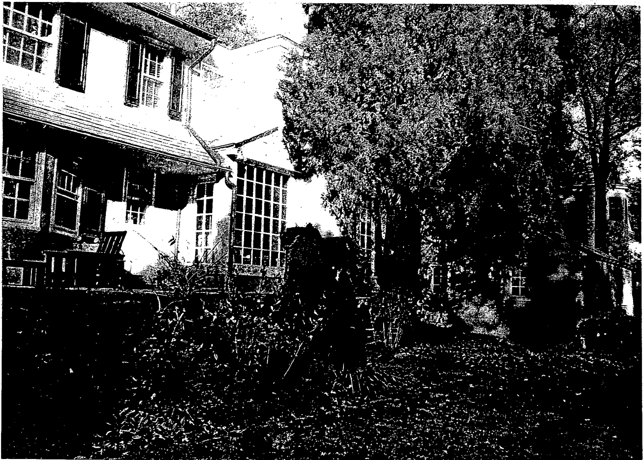
Detail, southeast corner of existing addition
