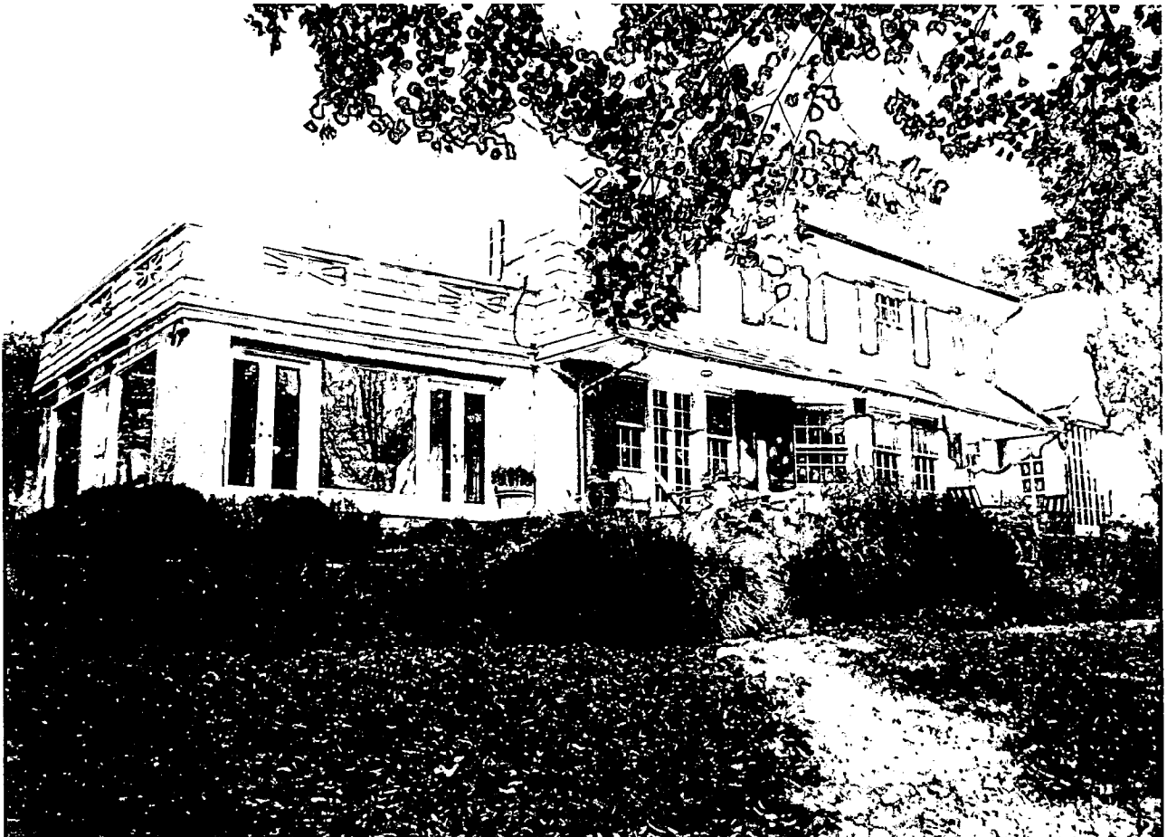
Rear (southwest) elevation from yard
