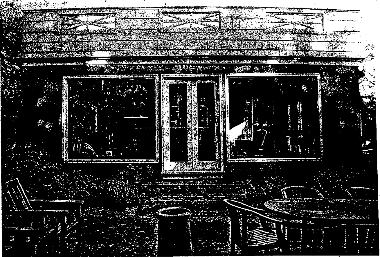
Detail, west elevation of one-story portion
