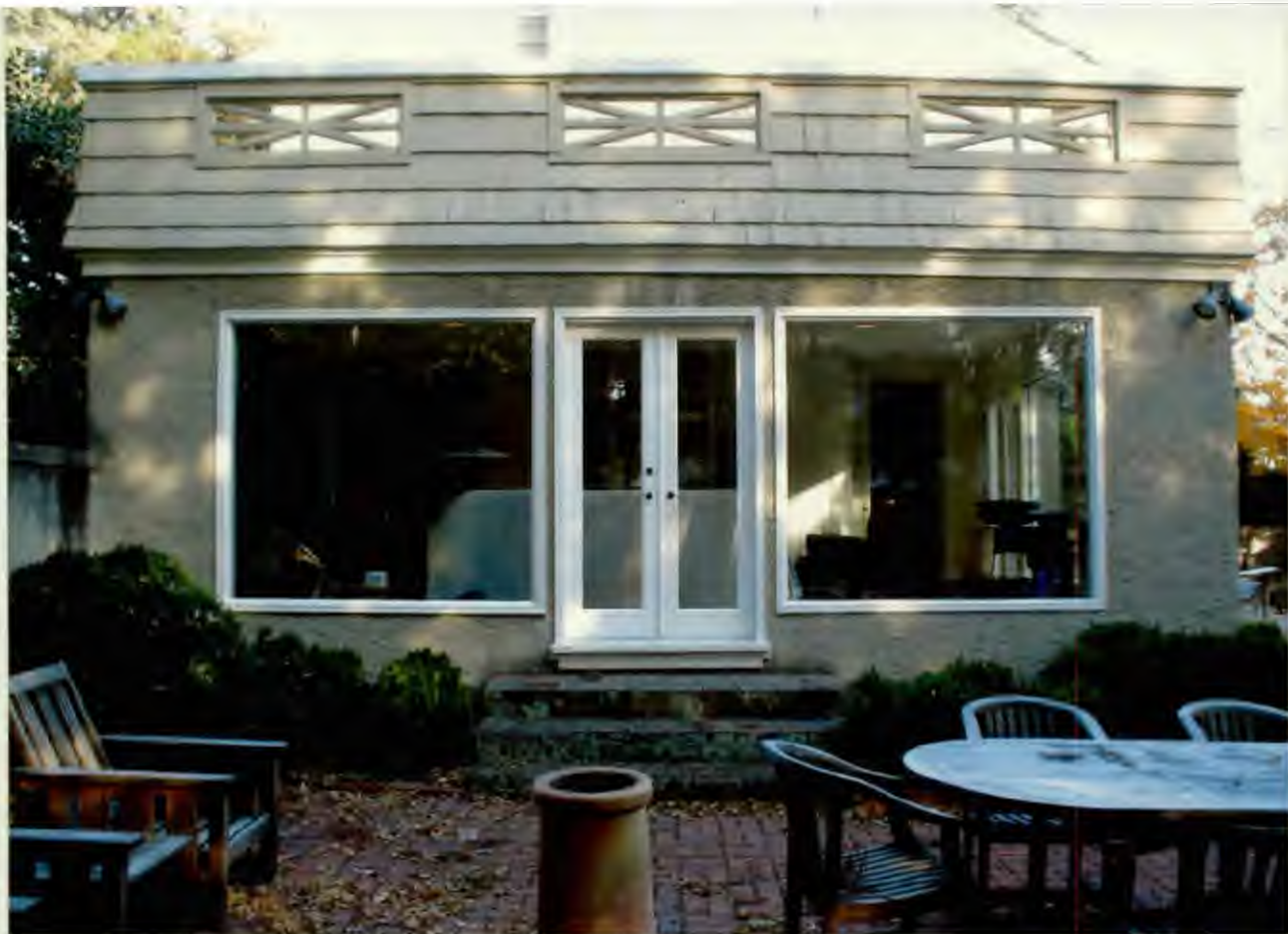
Detail, west elevation of one-story portion
