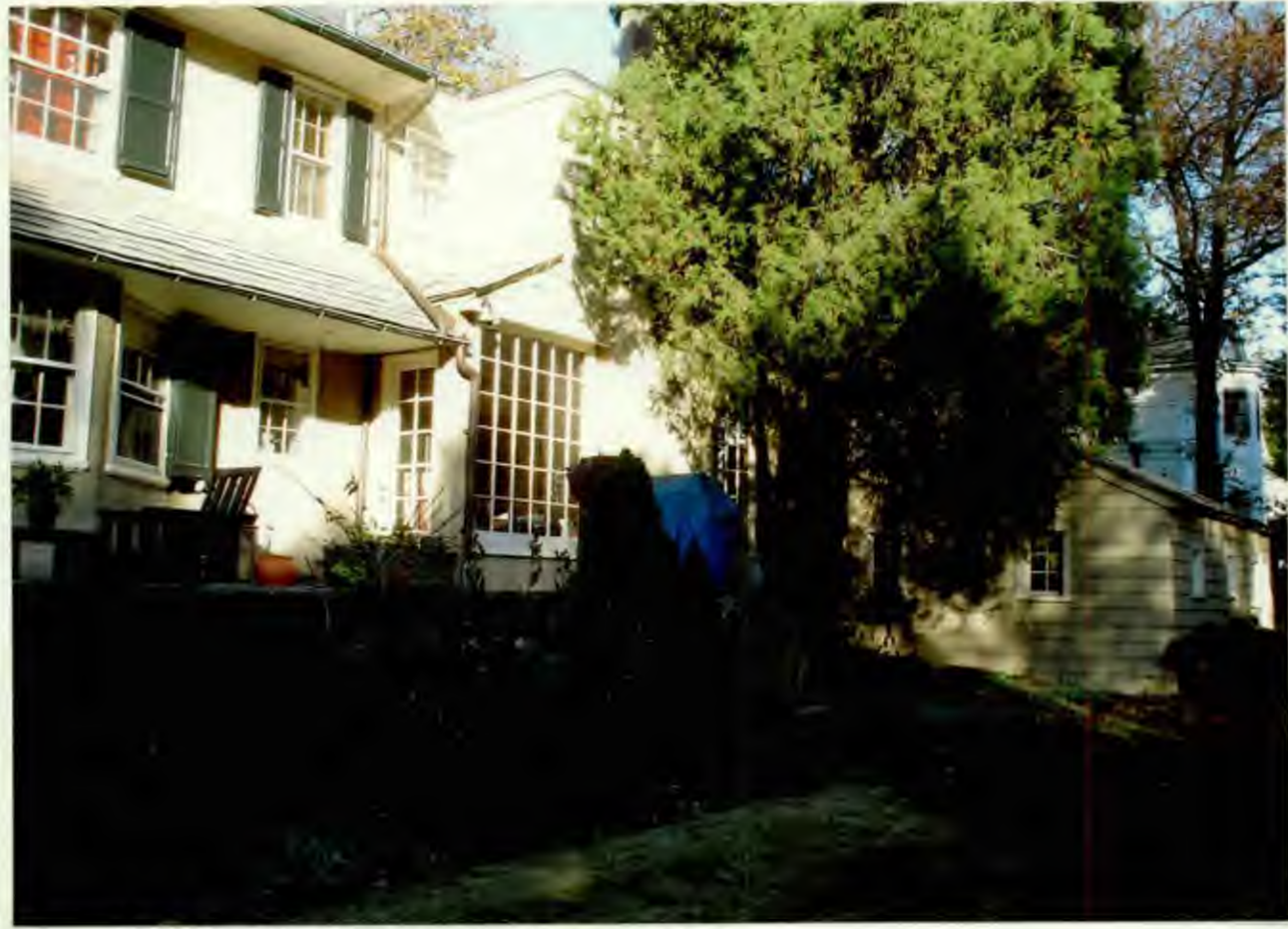
Detail, southeast corner of existing addition
