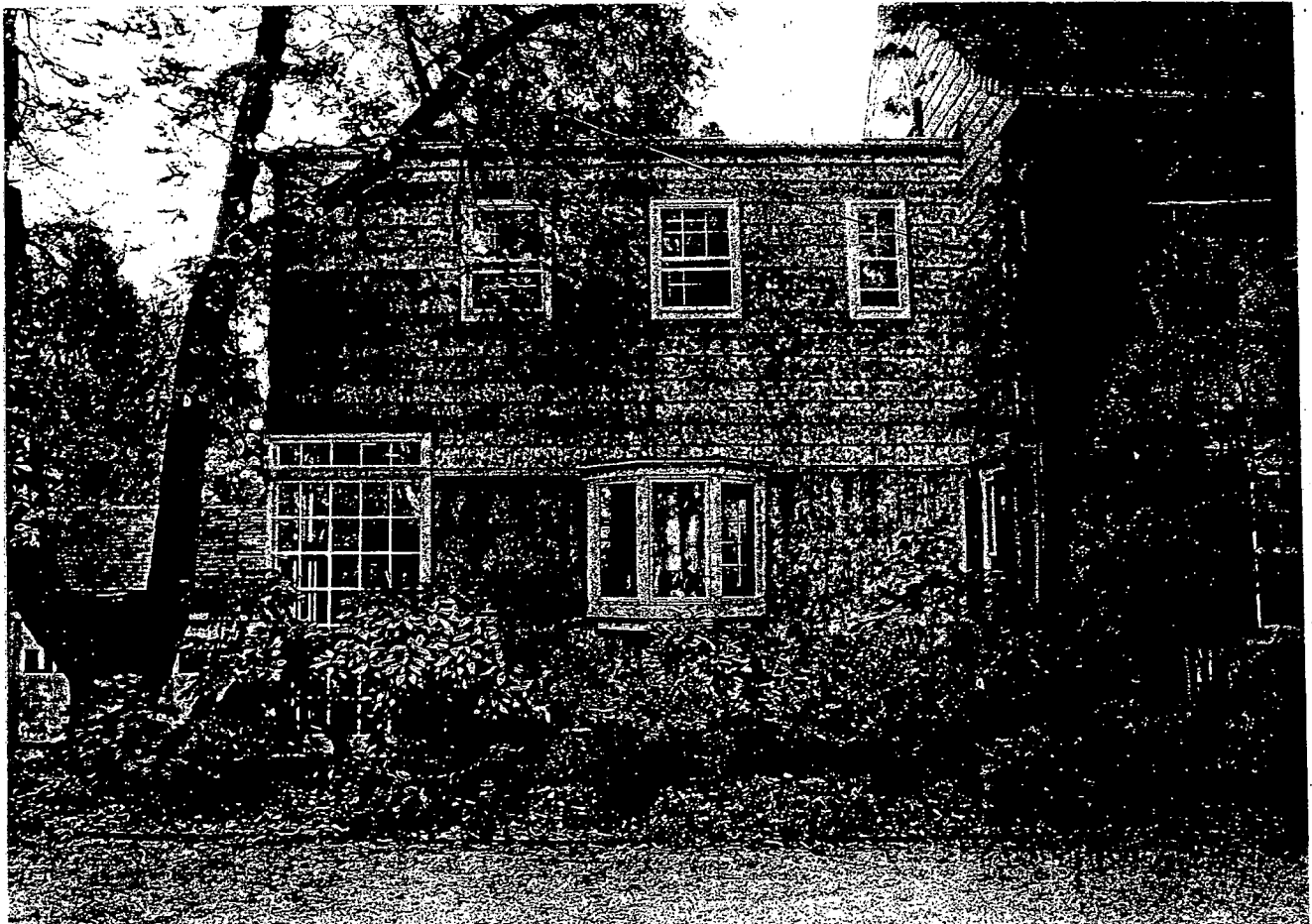
Detail, north elevation of existing addition
