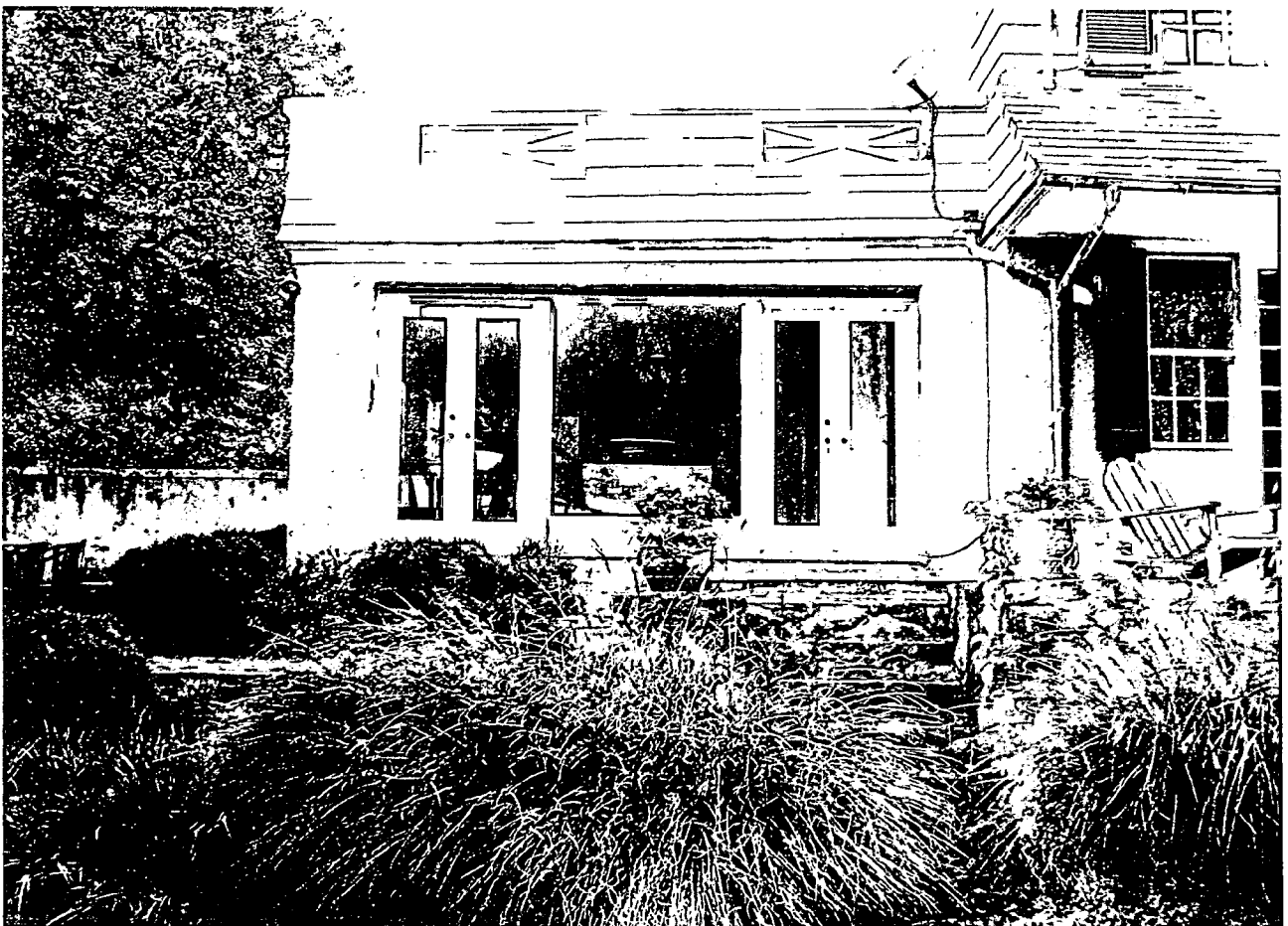
Detail, south elevation of existing one-story portion
