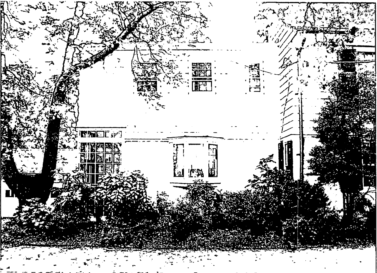
Detail, north elevation of existing addition
