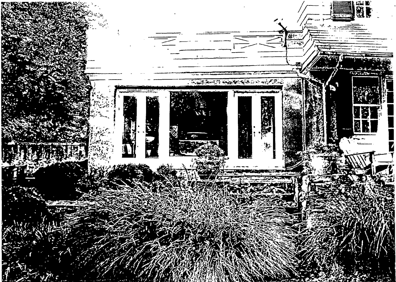
Detail, south elevation of existing one-story portion
