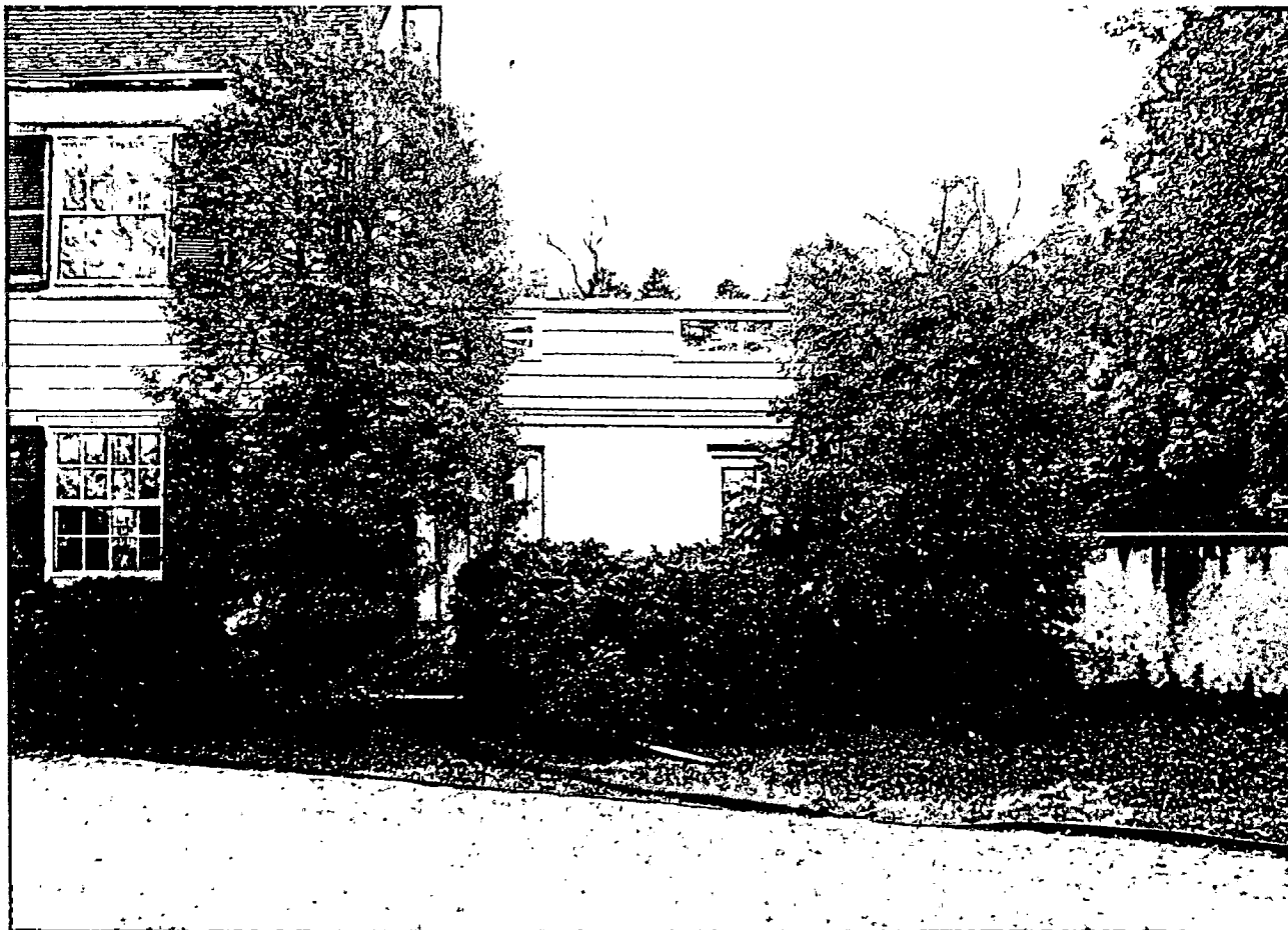
Detail, northwest corner one-story portion
