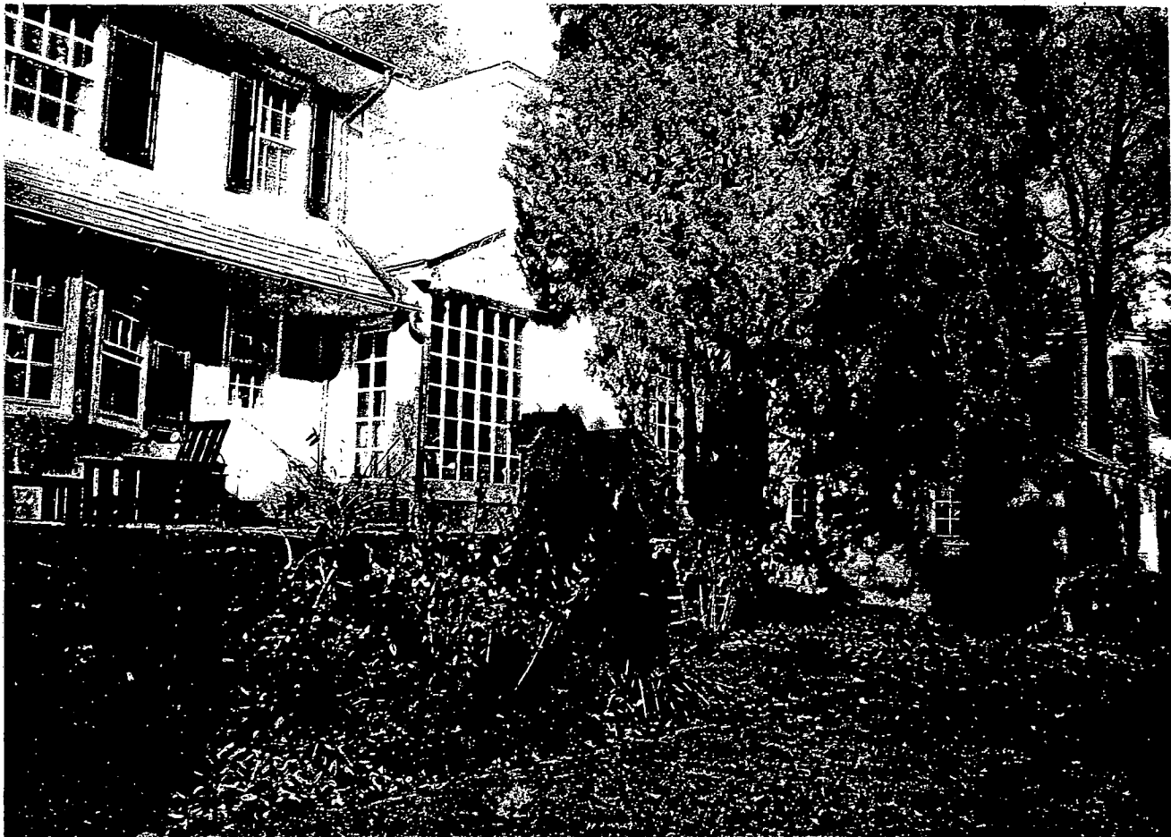
Detail, southeast corner of existing addition
