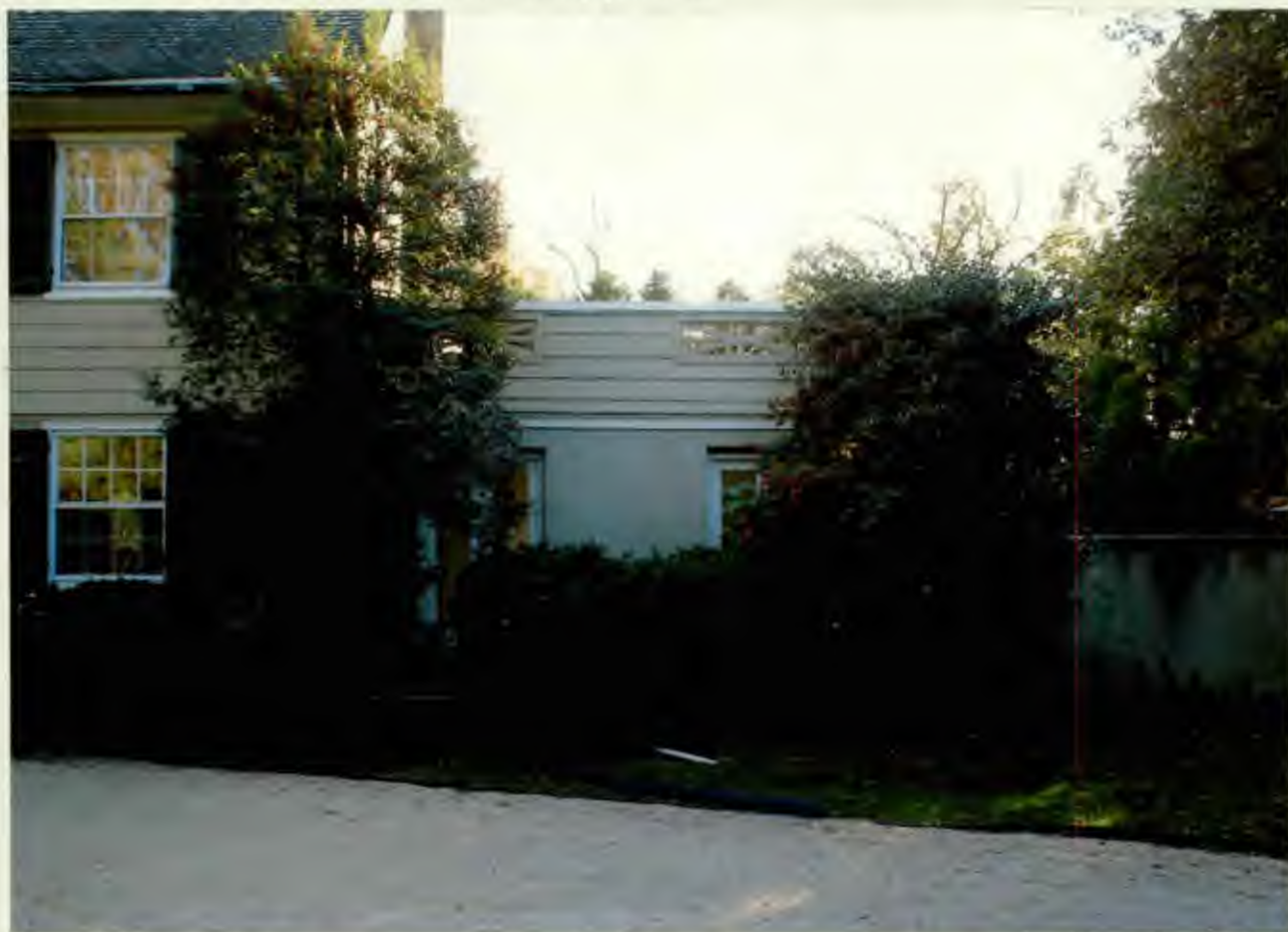
Detail, northwest corner one-story portion
