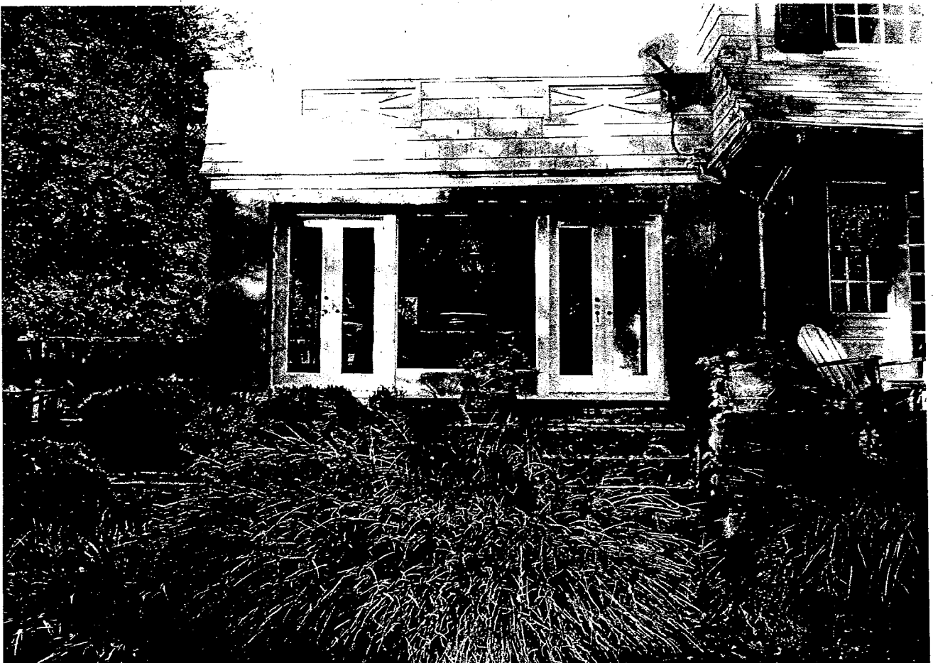
Detail, south elevation of existing one-story portion
