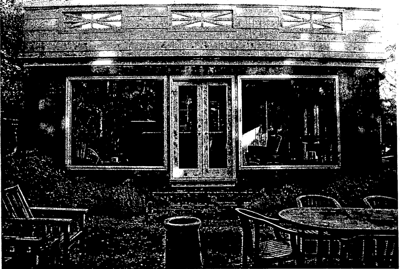
Detail, west elevation of one-story portion
