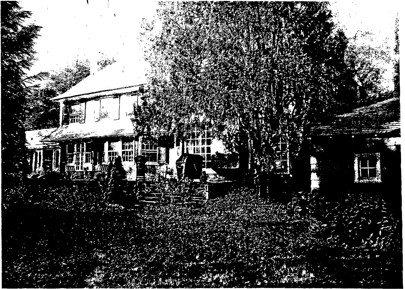
Rear (southeast) elevation from yard
