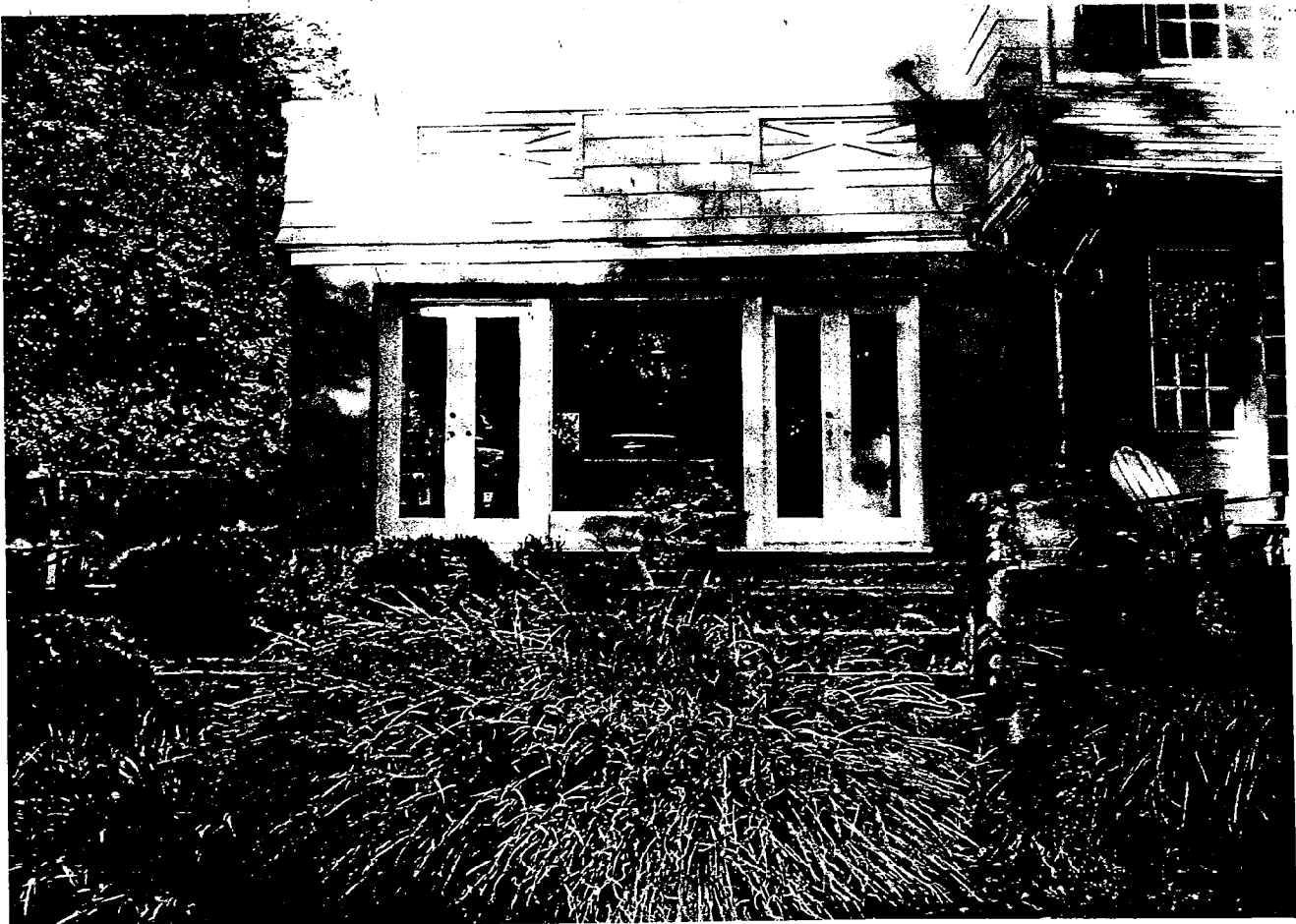
Detail, south elevation of existing one-story portion
