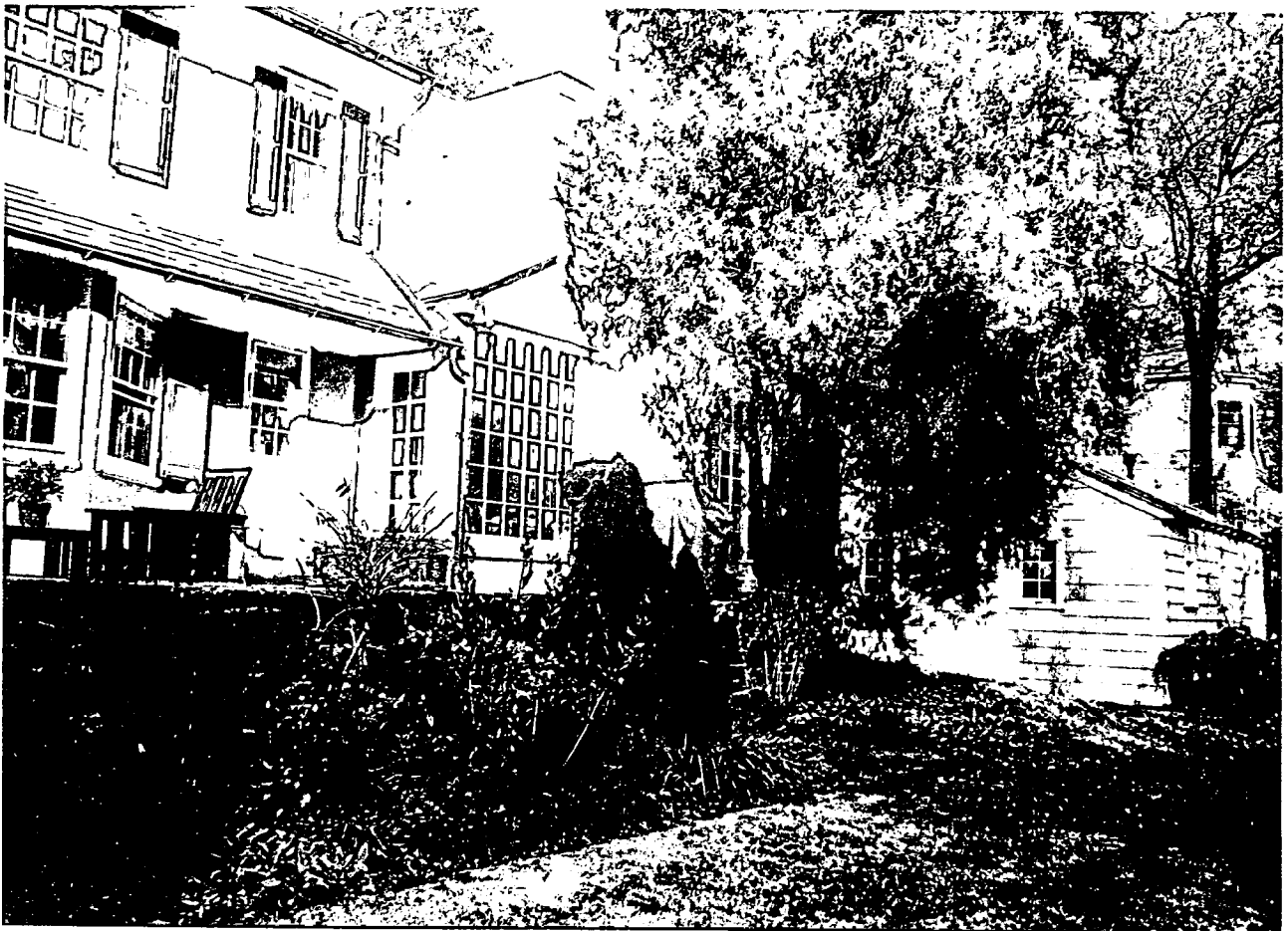
Detail, southeast corner of existing addition
