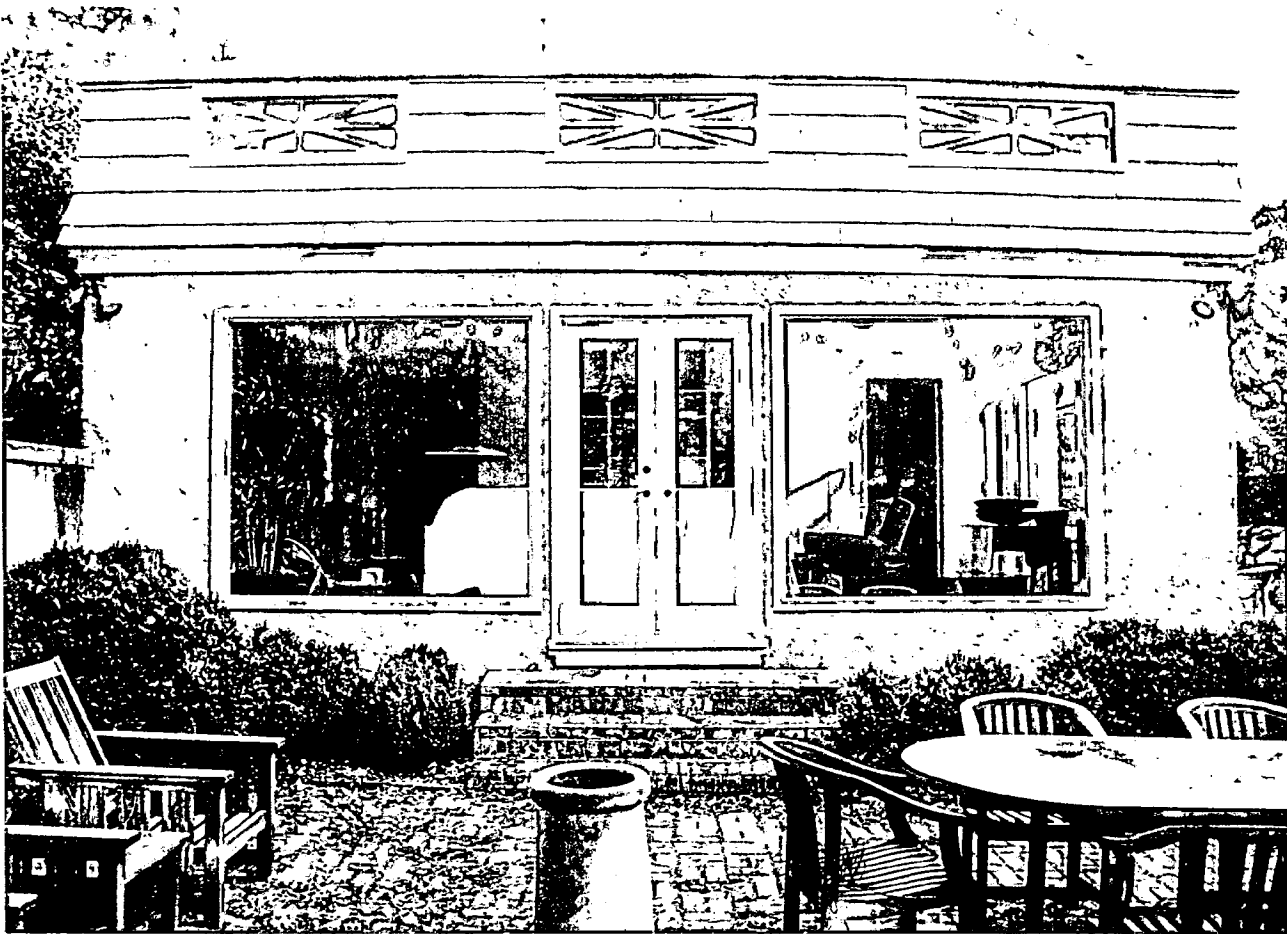
Detail, west elevation of one-story portion
