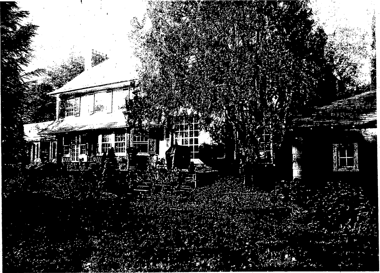
Rear (southeast) elevation from yard
