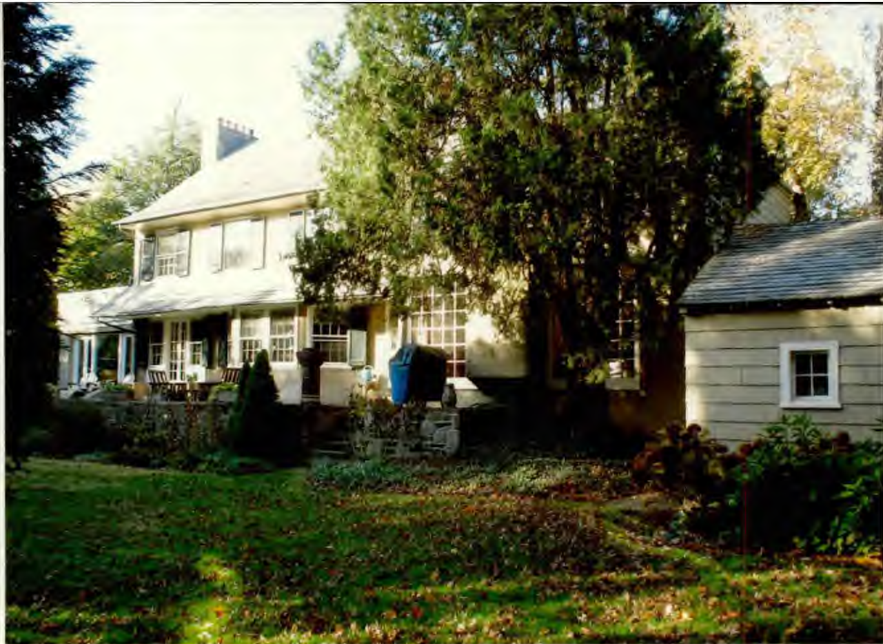
Rear (southeast) elevation from yard
