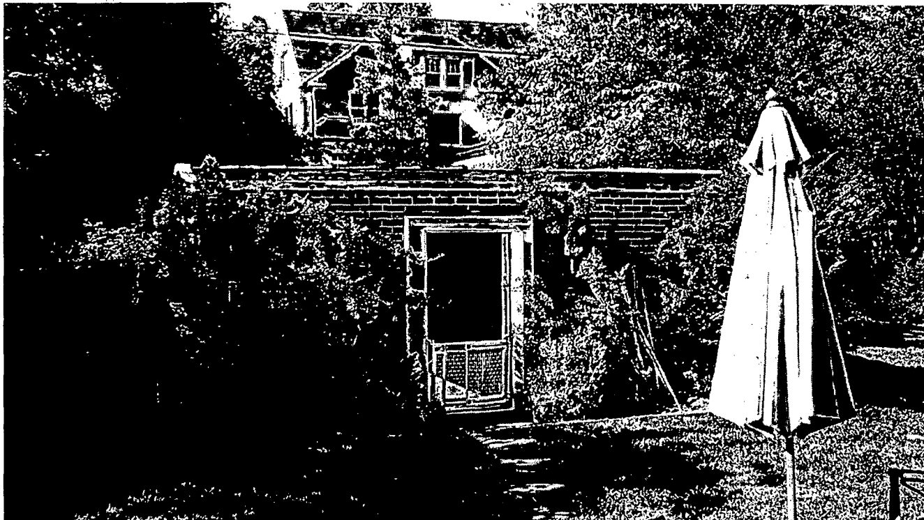
GARAGE - VIEW FROM MAIN HOUSE
