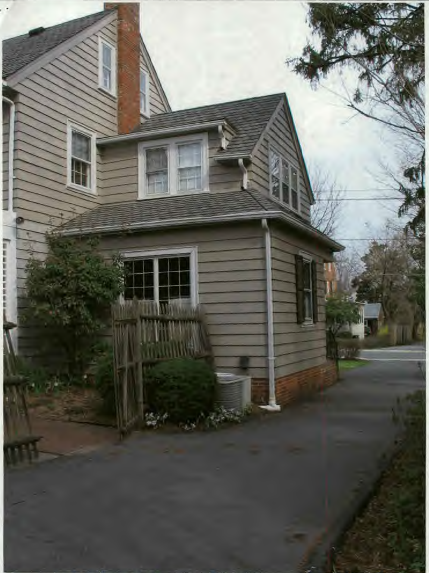
SILBER RESIDENCE: EXISTING PROPERTY 3720 BRADLEY LN. CONDITION
