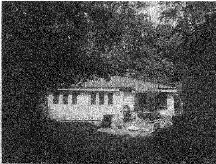
Garage and Rear Driveway Doors to be Replaced 2201 Salisbury Rd.
