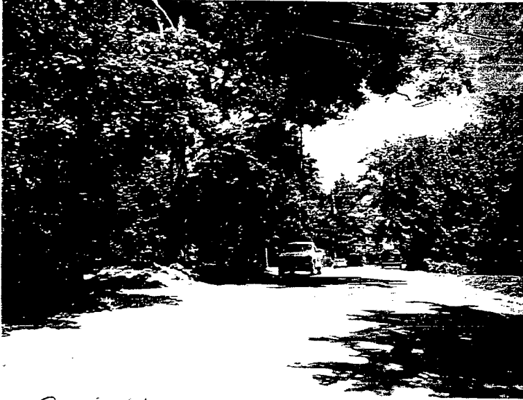
East View Streetscape 2201 Salisbury Road
