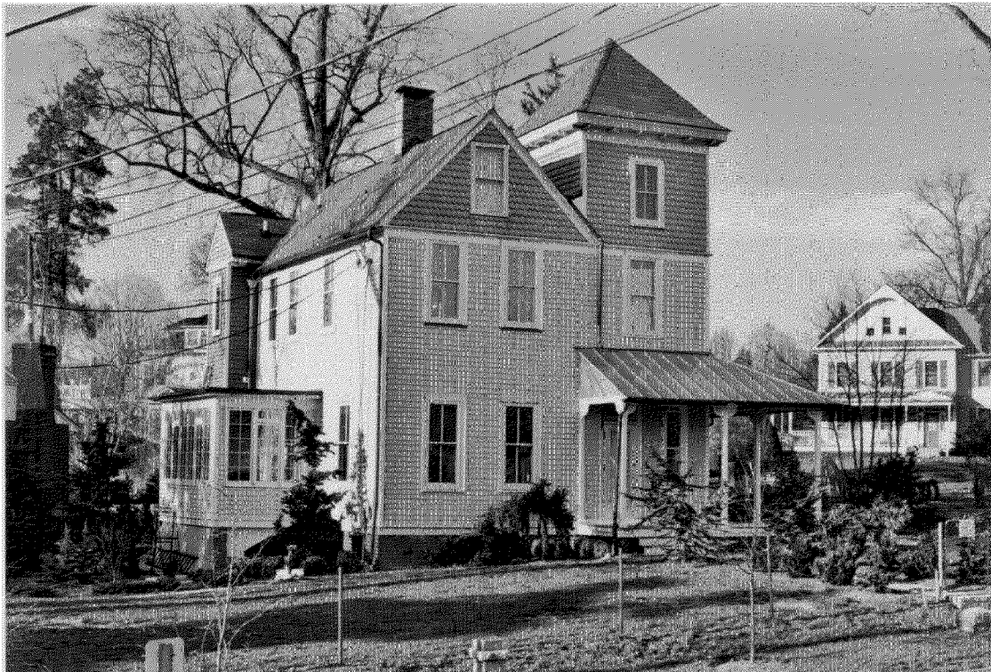
Front facade - front view of subgreenhouse and existing gutter/gusset
