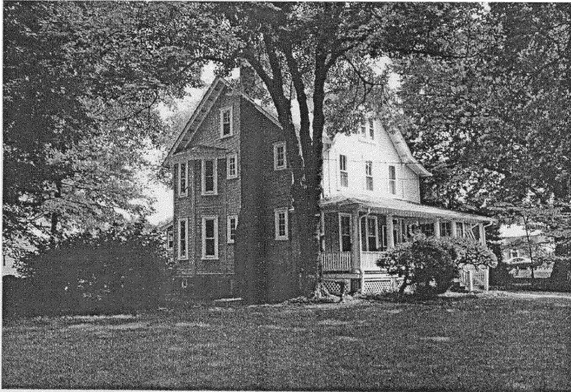
LEFT FRONT (VIEWED FROM RIGHT-OF-WAY)
