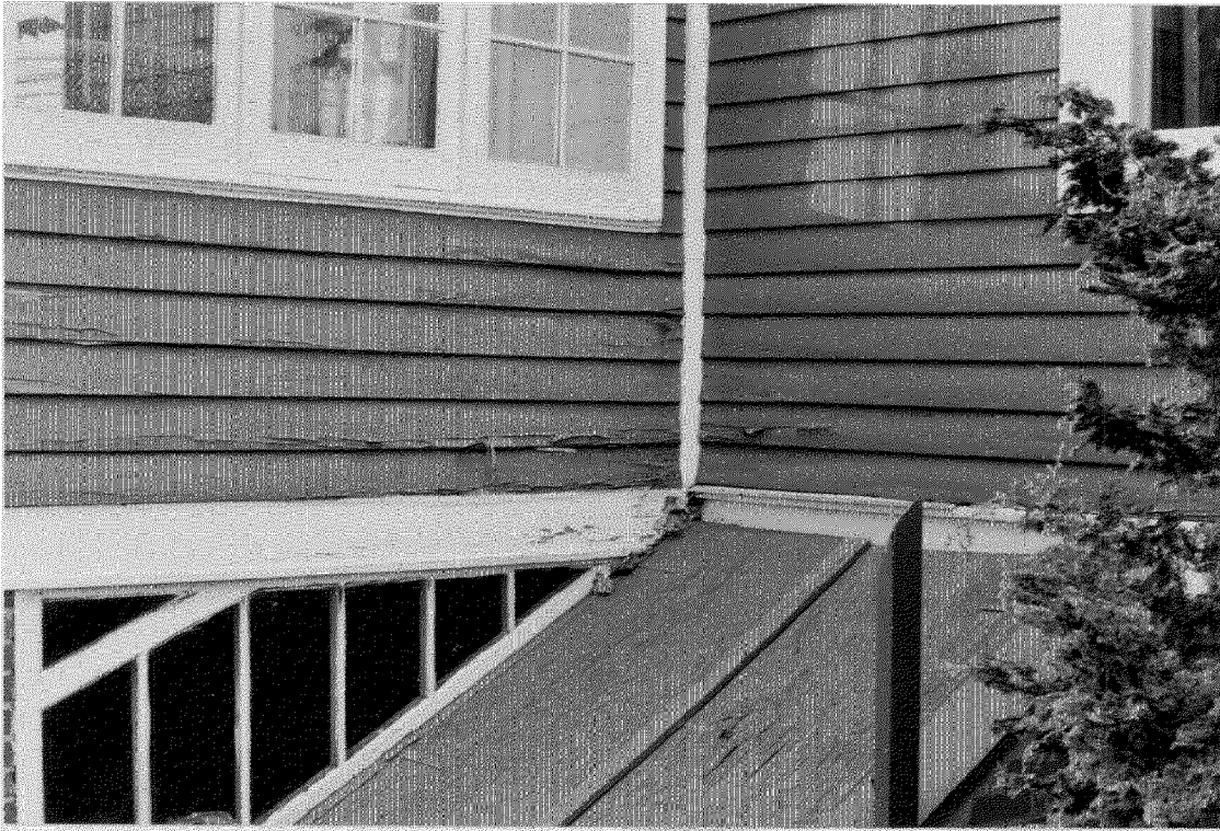
Detail: Basement entrance doors / corner house wall + greenhouse
