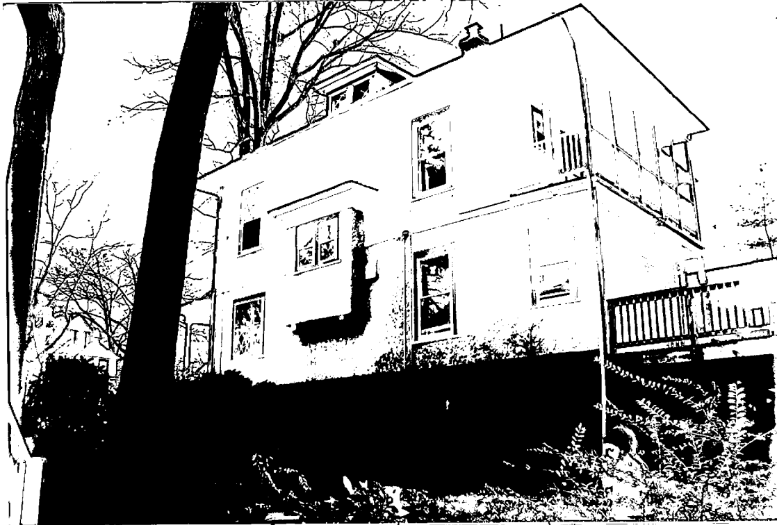
Detail: side facade (east side)
