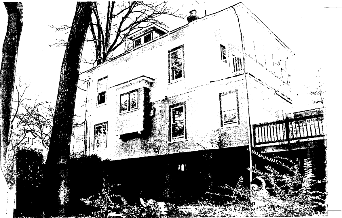
Detail: side facade (east side)
