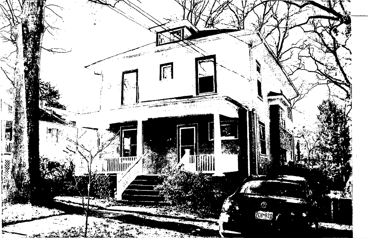
Detail: front facade from public right-of-way (south)
