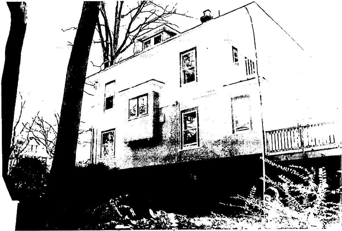
Detail: side facade (east side)
