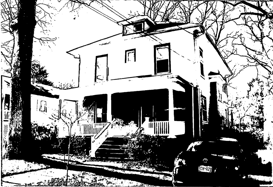
Detail: front facade from public right of way (south)
