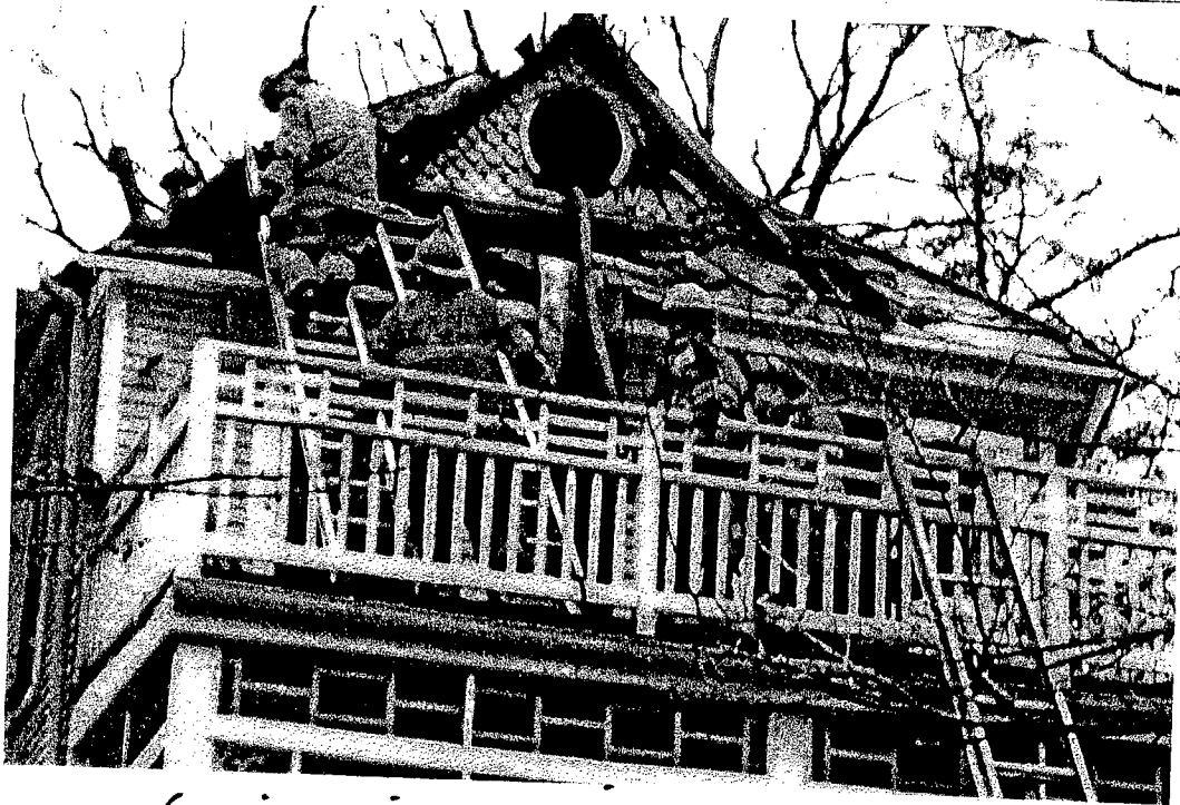
REAR (DURING FIRE) SHOWING DORMER
