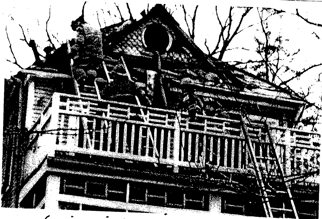
REAR (DURING FIRE) SHOWING DORMER
