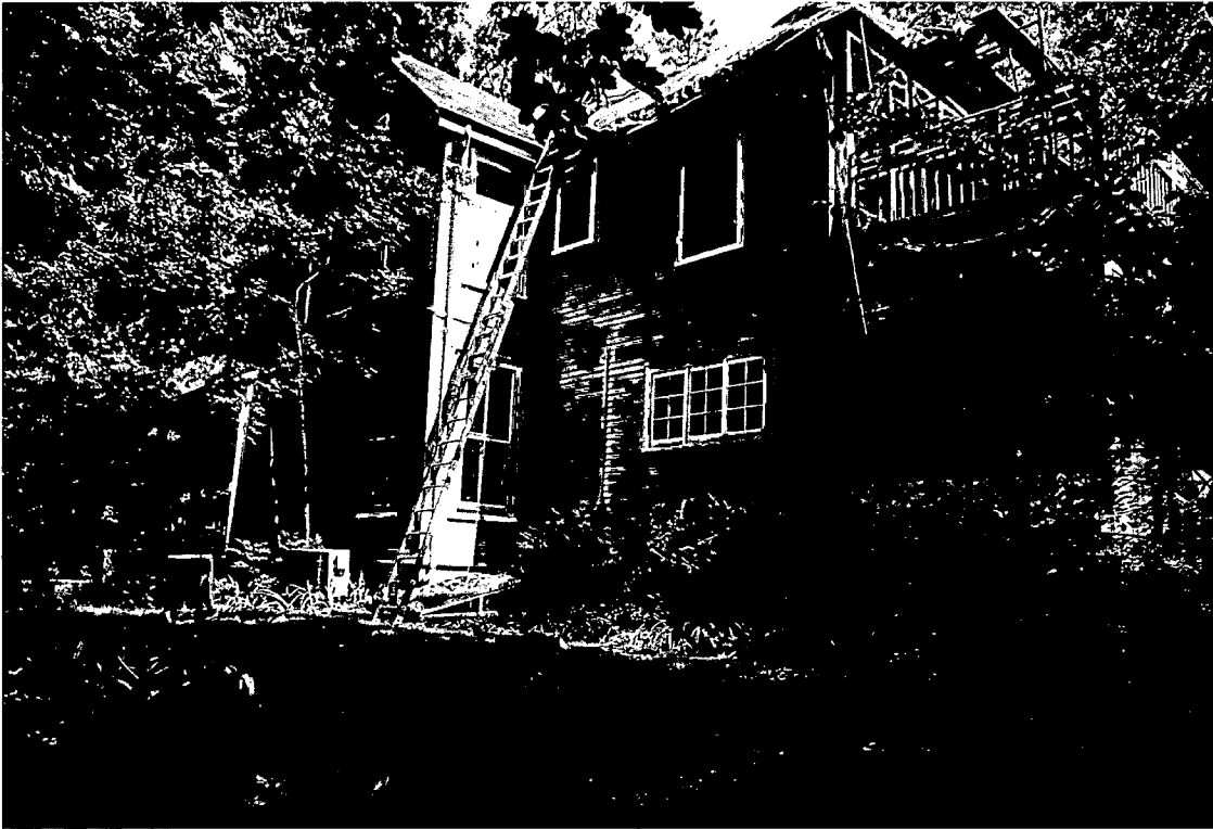
7315 Piney Branch Rd, South Elevation.
