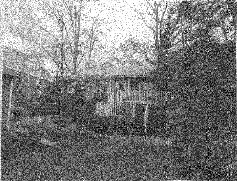
Detail: Rear yard view of previous addition & deck to be removed
