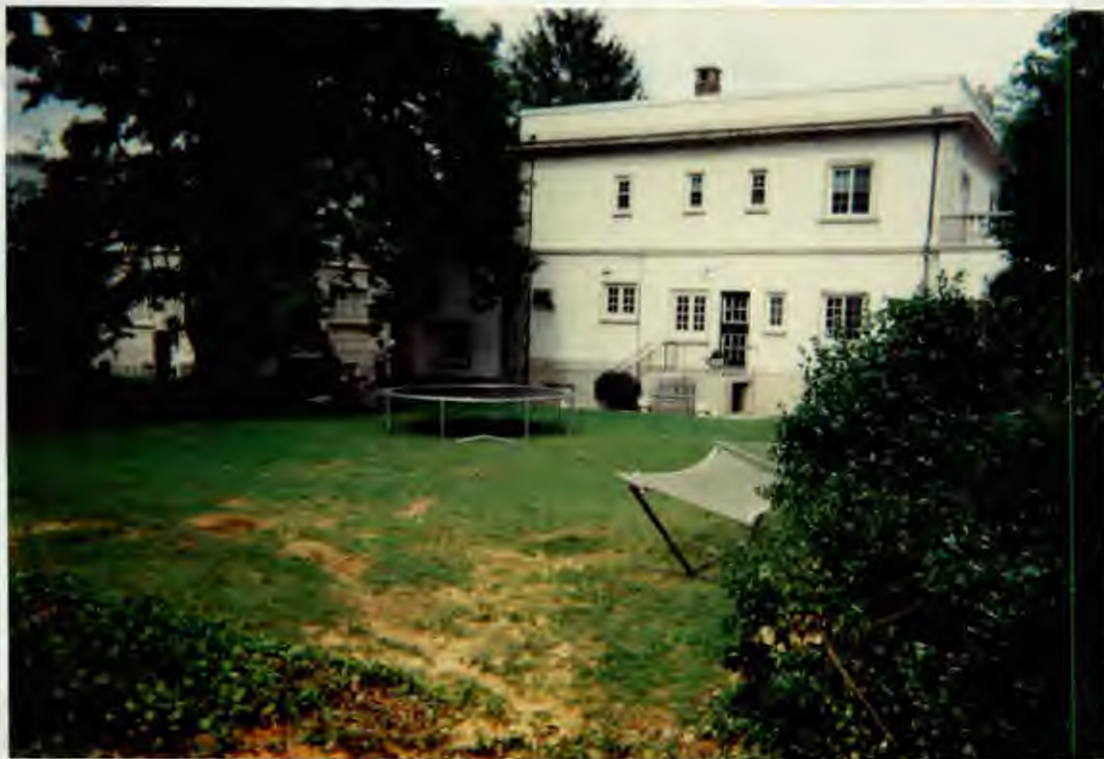
↑ VIEW FROM LEFT REAR OF PROPERTY FACING THE REAR OF THE RESIDENCE.
