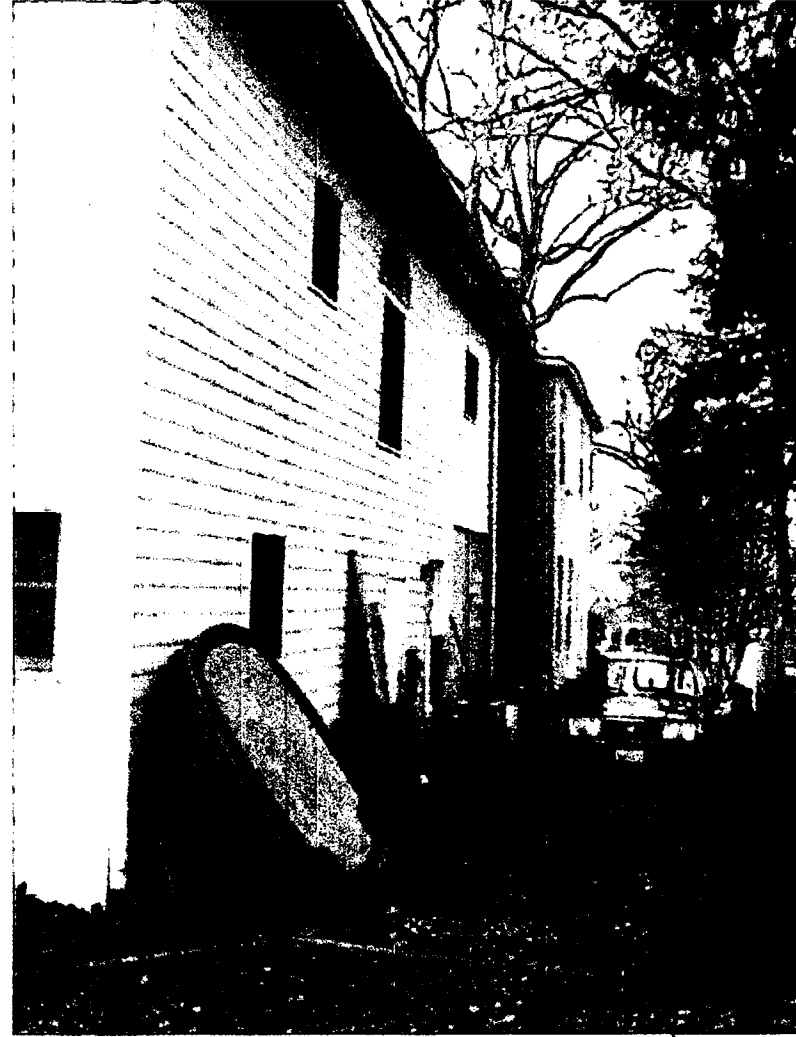
North Side Elevation (from Northeast Corner)
