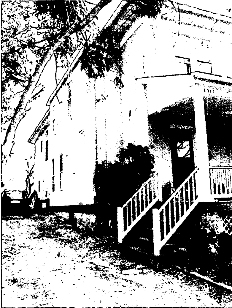
North Side Elevation (from Northwest Corner)
