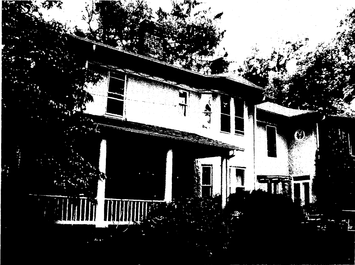
South Side View Proposed Addition at First Floor in Recessed Bay and Screened Porch located to right by Holly Trees
