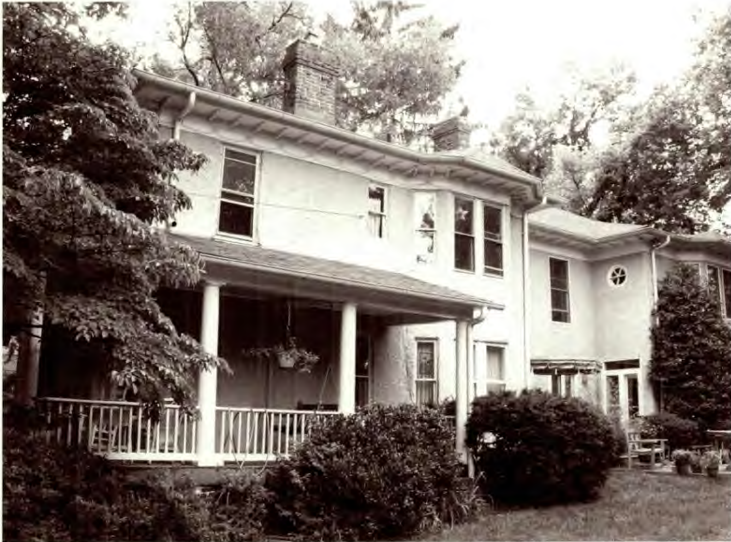
South Side View Proposed Addition at First Floor in Recessed Bay and Screened Porch located to right by Holly Trees
