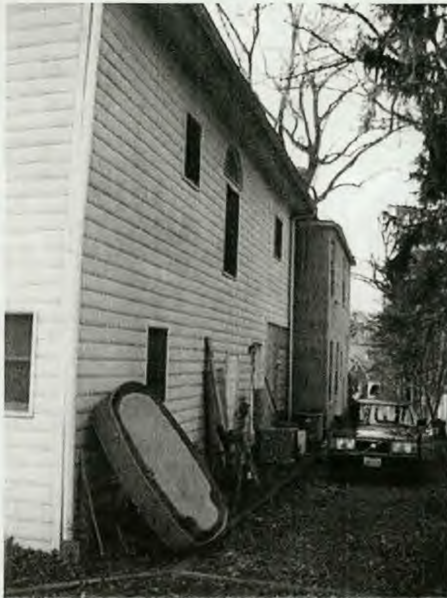
North Side View - Northeast Corner Proposed Rear Entry located at Center Door
