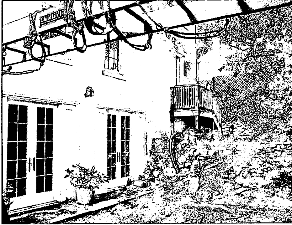
basement level of house (formerly a garage)
