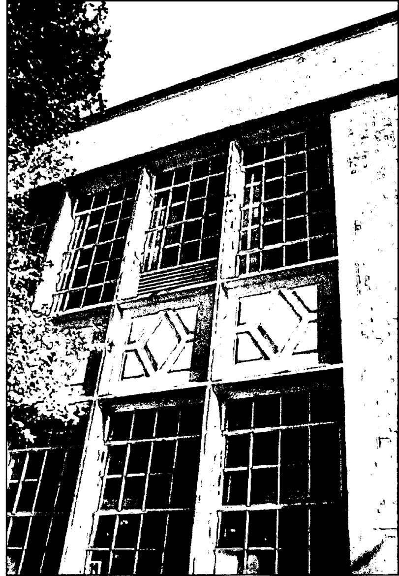
2 Limestone Window Details at West Wing, West Elevation
