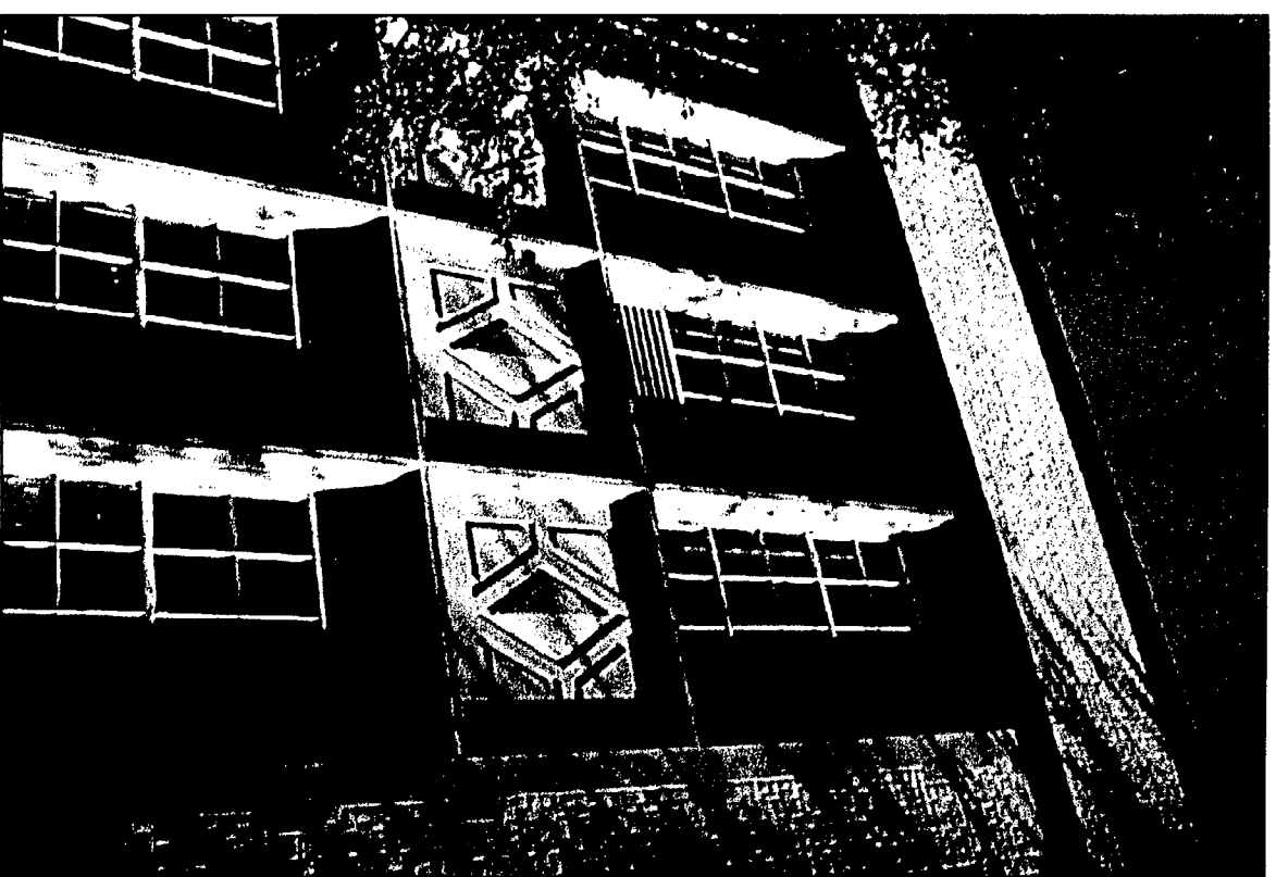
2 Limestone Window Details at West Wing, West Elevation
