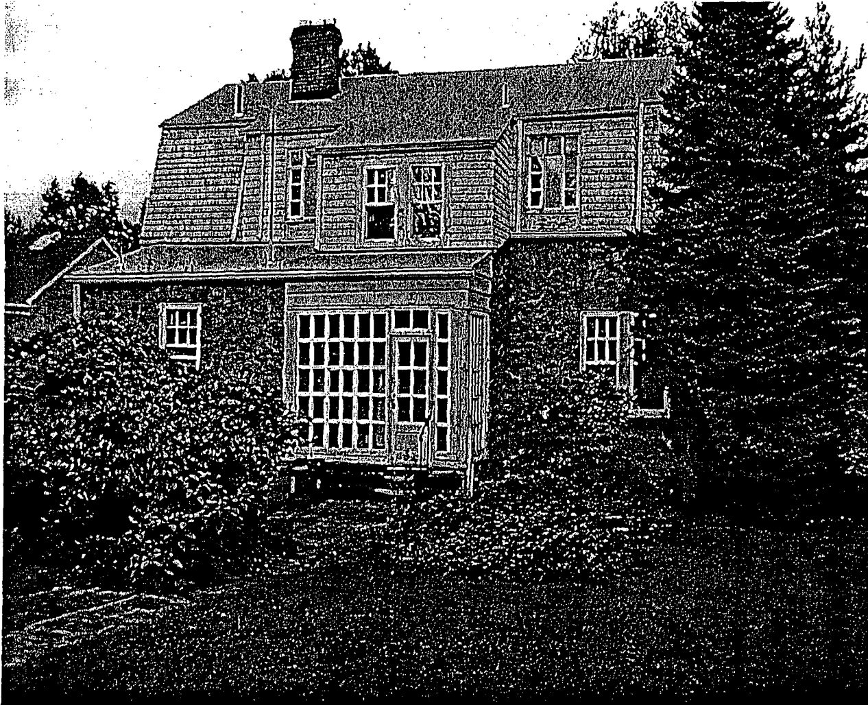
5004 River Road Rear Elevation
