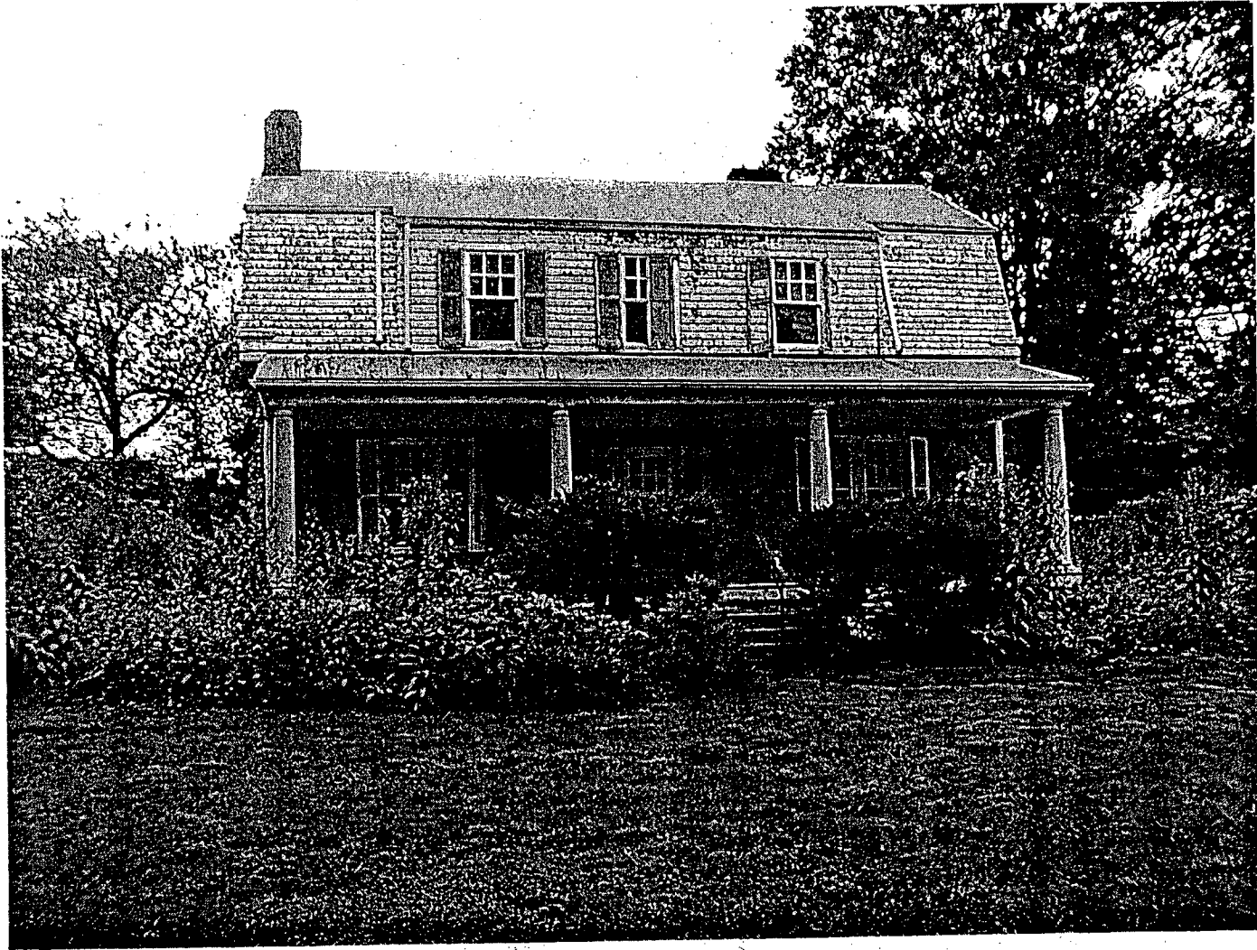
5004 River Road Front Elevation
