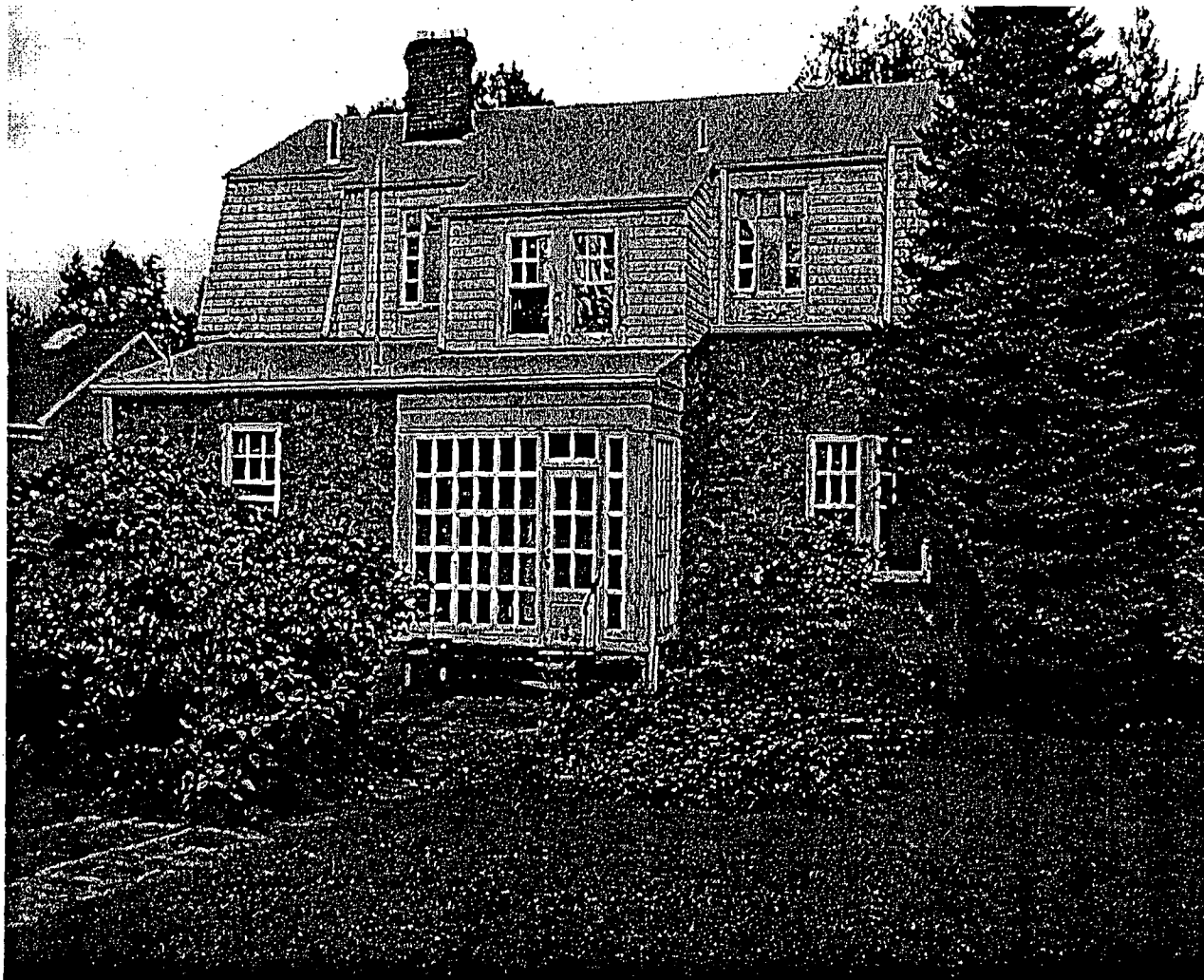
5004 River Road Rear Elevation
