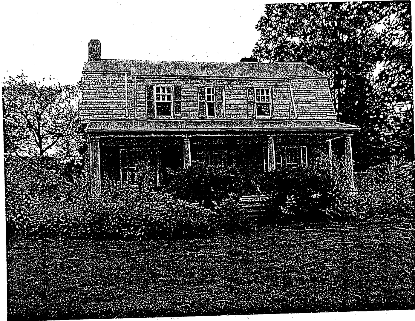
5004 River Road Front Elevation
