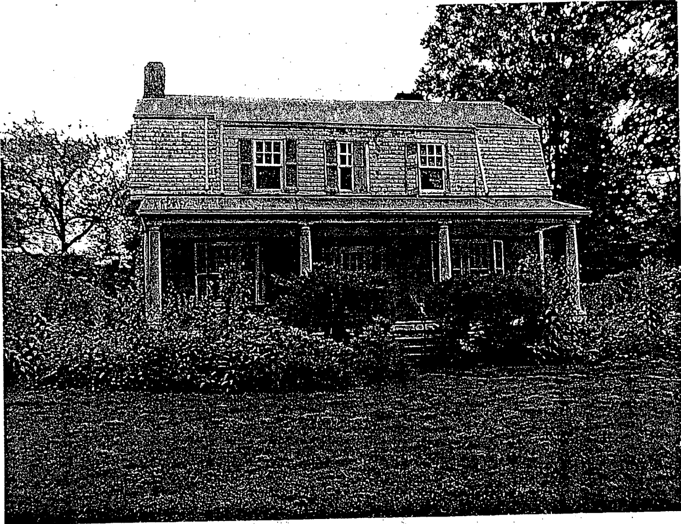
5004 River Road Front Elevation
