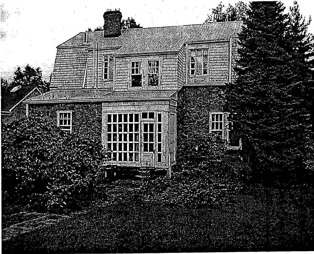
5004 River Road Rear Elevation
