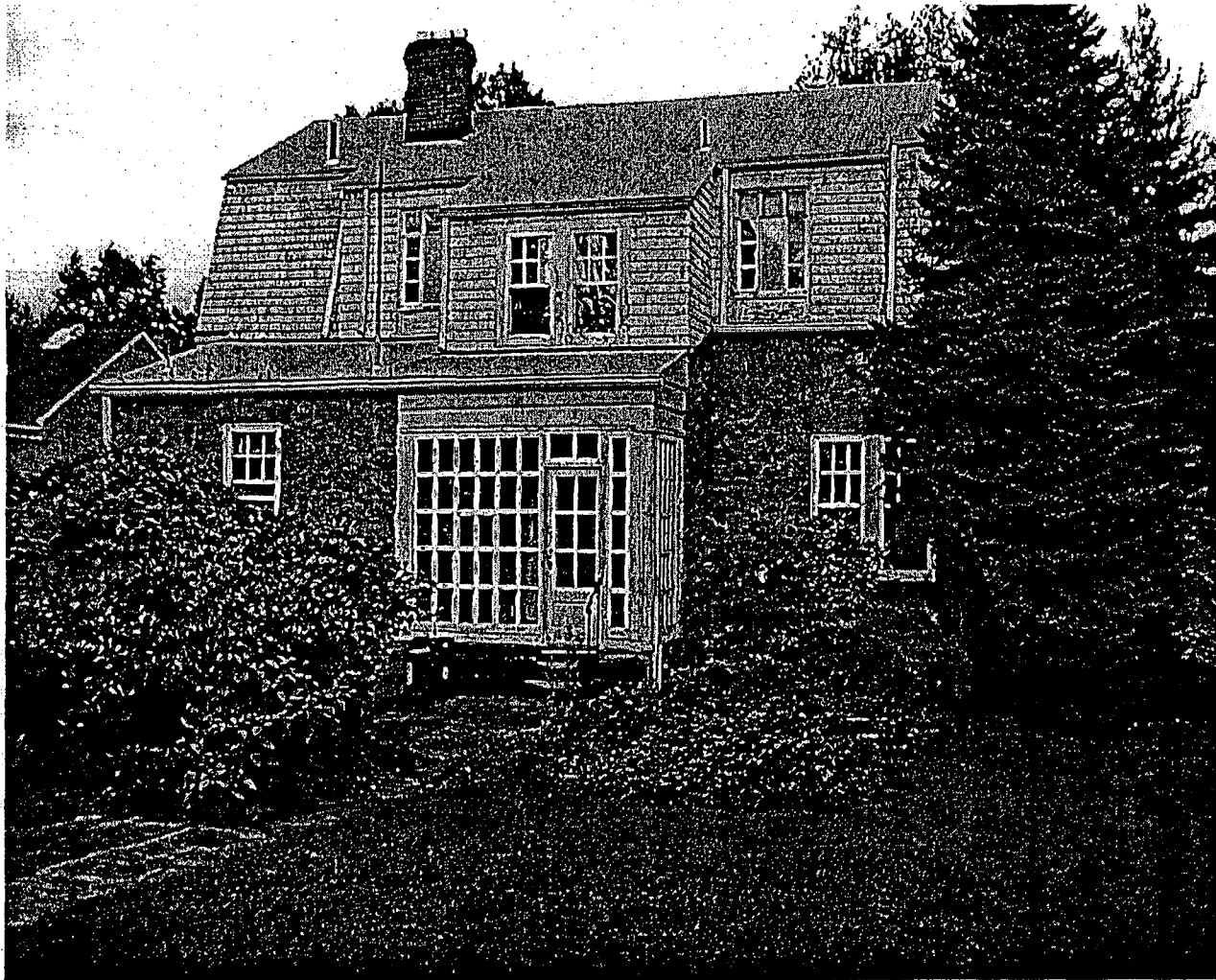
5004 River Road Rear Elevation
