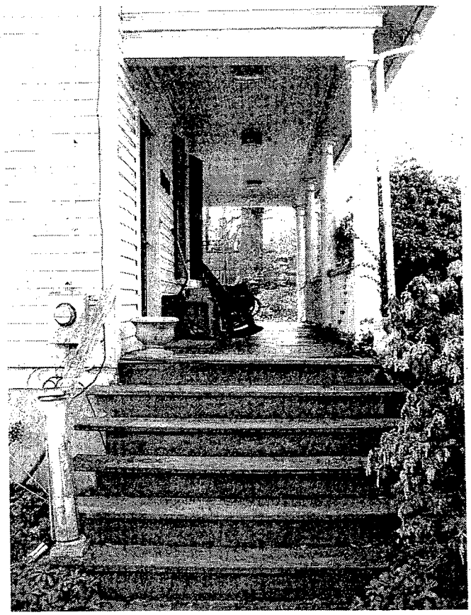
View of front porch from east
