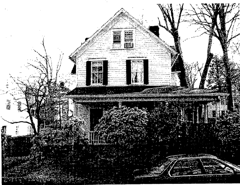
View of house from north
