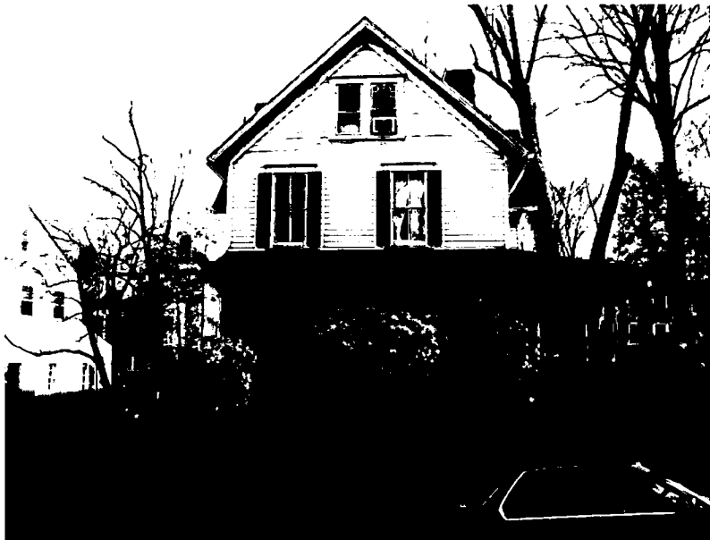
View of house from north
