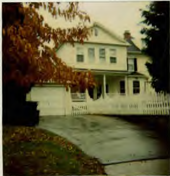
LEFT SIDE OF HOUSE FROM DARKEITH ST
