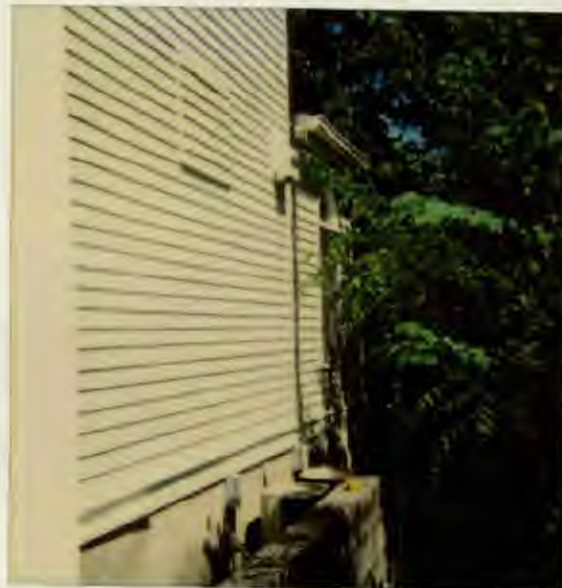
RIGHT SIDE OF HOUSE LOCATION OF 2ND FLOOR ADDITION
