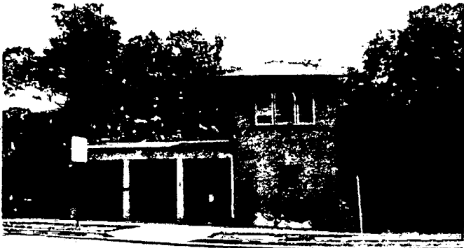
North façade existing- posts, flat roof Tower roof
