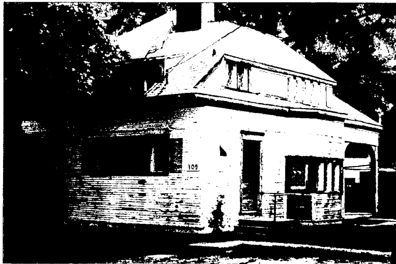
South west roof line and corner of dormer to be restored.
