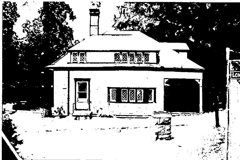
Photo shows more of south roof and walkways in the yard. Can see location of the Pagoda to the Northwest.
