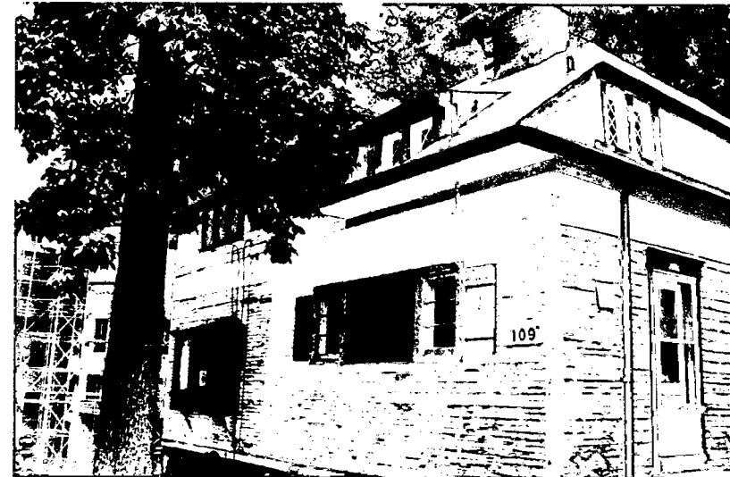
Hickory tree located at west façade. Tree is now dying due to public underground utility work done running parallel to the Linden La. Between the tree and the sidewalk.
