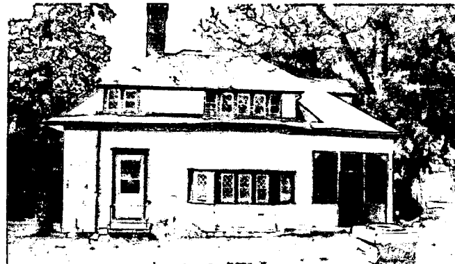
South facade- roof line and land area. Stone pillar once staged a statue on the school grounds.
