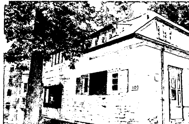
Hickory tree located at west facade. Tree is now dying due to public underground utility work done running parallel to the Linden La. Between the tree and the sidewalk.
