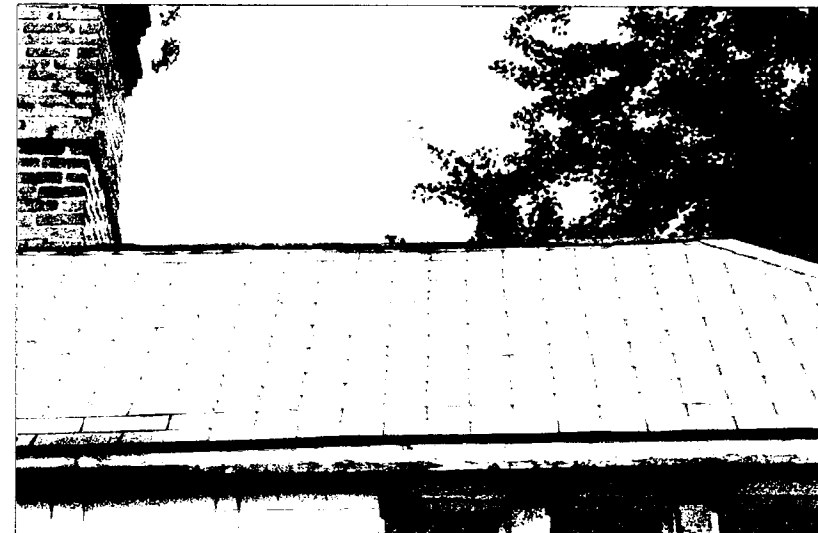
More of the existing roof, missing gutters, and fascia board in need of repair.
