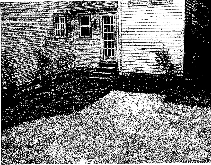
Photo 6: Back steps at proposed patio area, low drainage point
