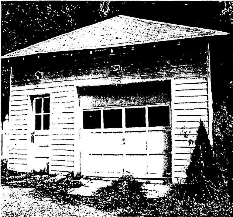
Current Garage Door. Note deterioration at bottom.
