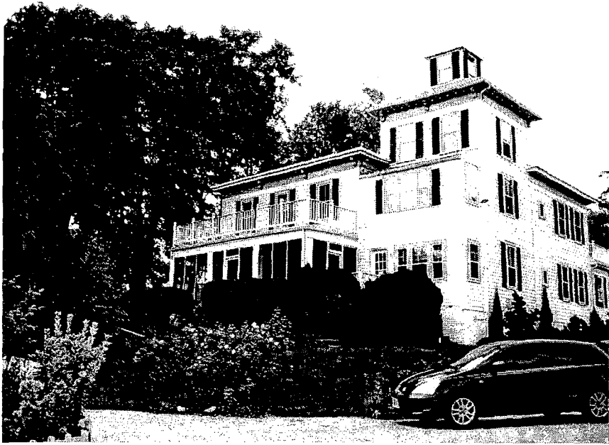
Photo 10: Front of house from Warren Court
