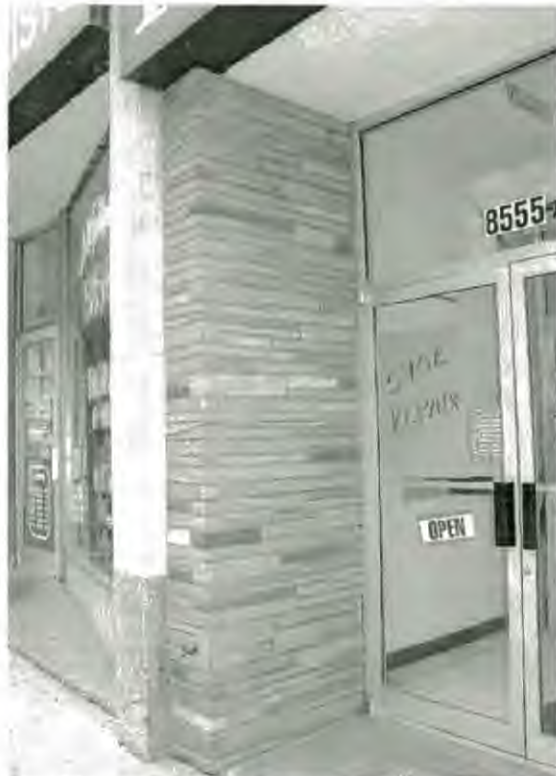
Non-original PermaStone wall surface
