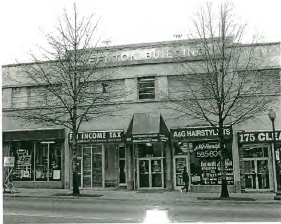
Main entrance on Fenton Street
