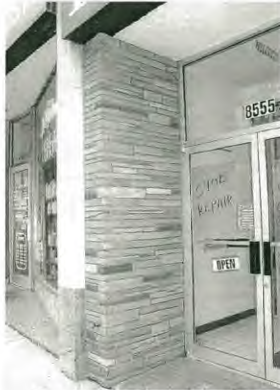
Non-original PermaStone wall surface
