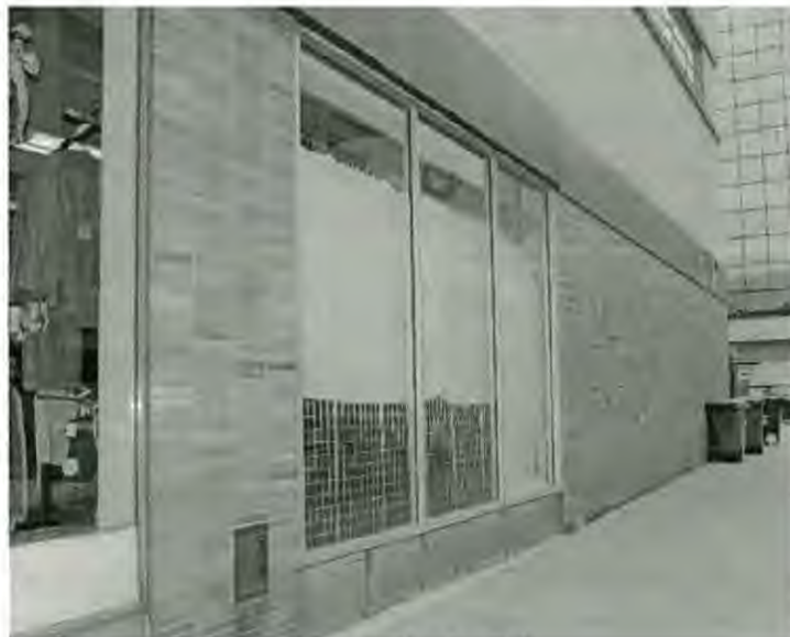
View on Roeder Rd.
