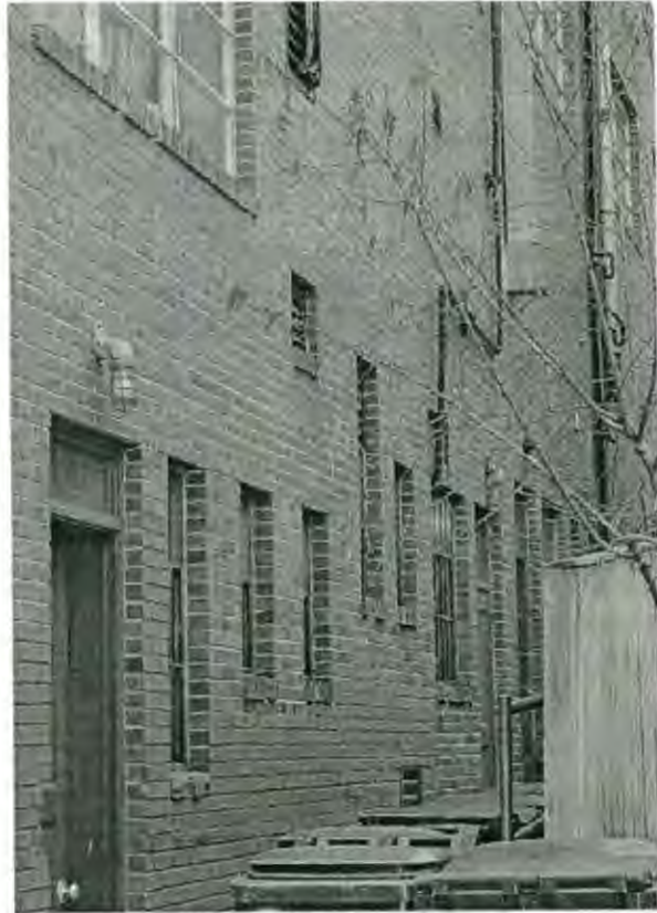
Back side of building along alley
