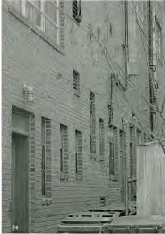
Back side of building along alley
