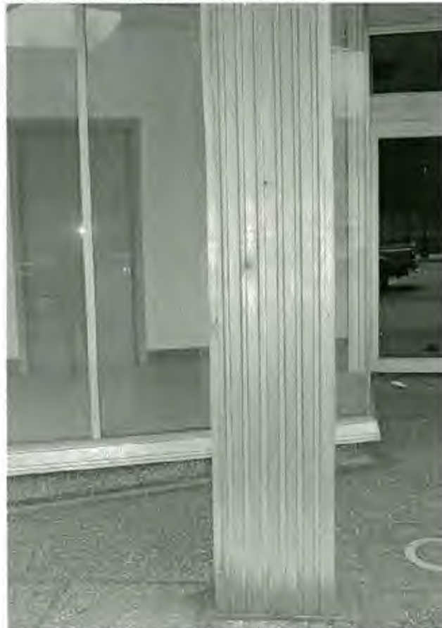
Detail of aluminum encased freestanding column
