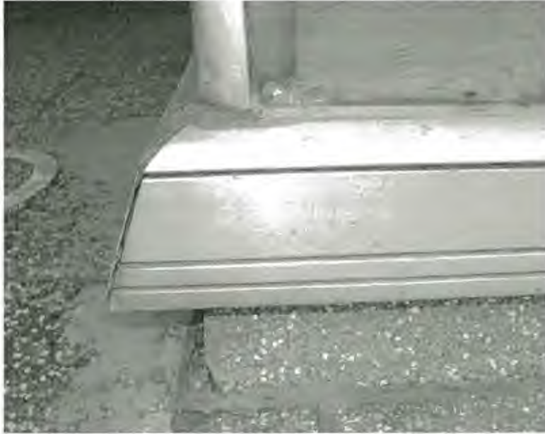
Detail of etched aluminum storefront system at Crawford Clothes
