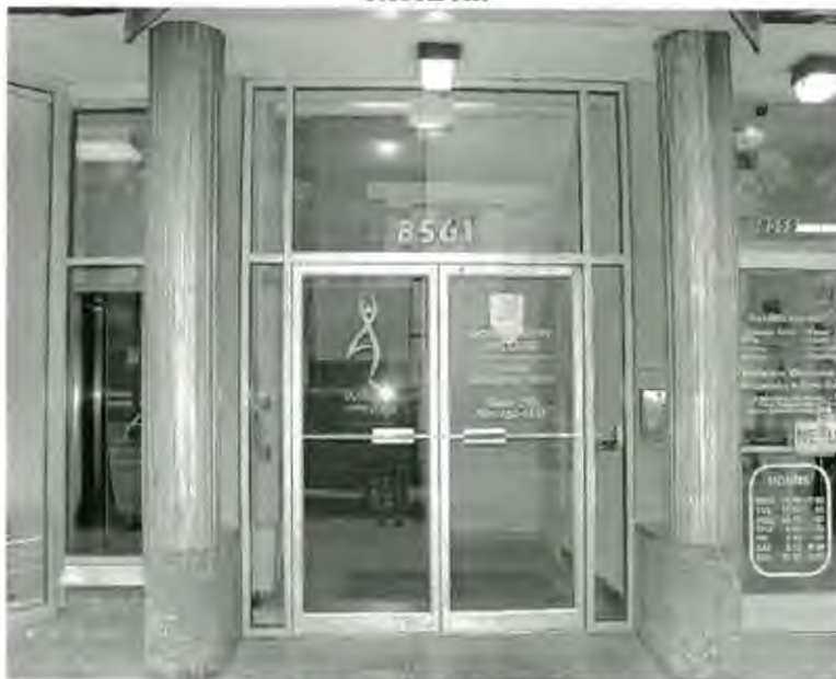
Main Entrance on Fenton Street
