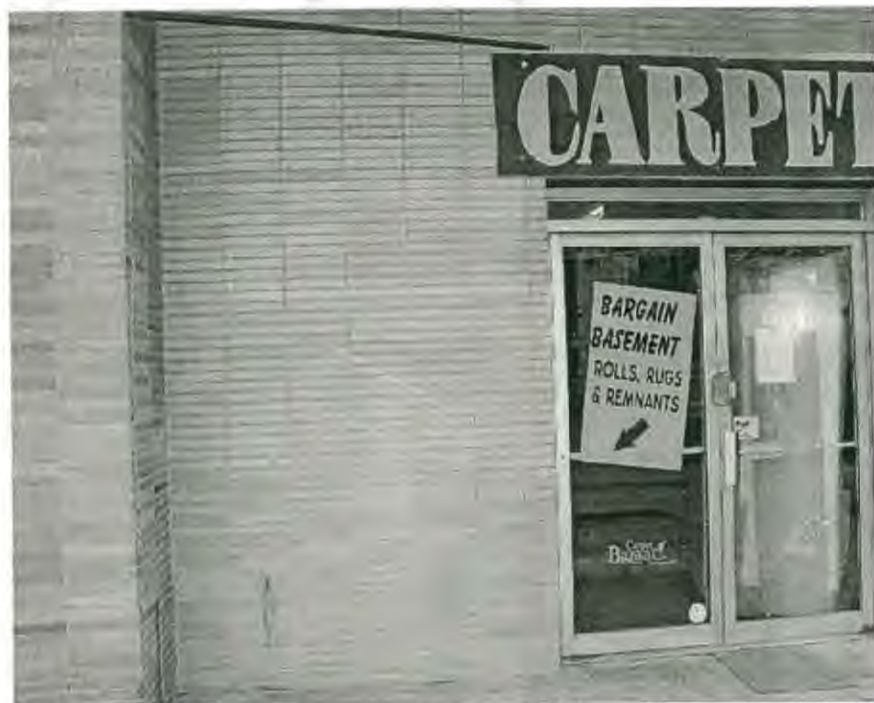
Wall of stretcher course iron-spot brick masonry
