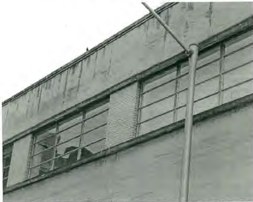
View of brushed aluminum ribbon windows on second story
