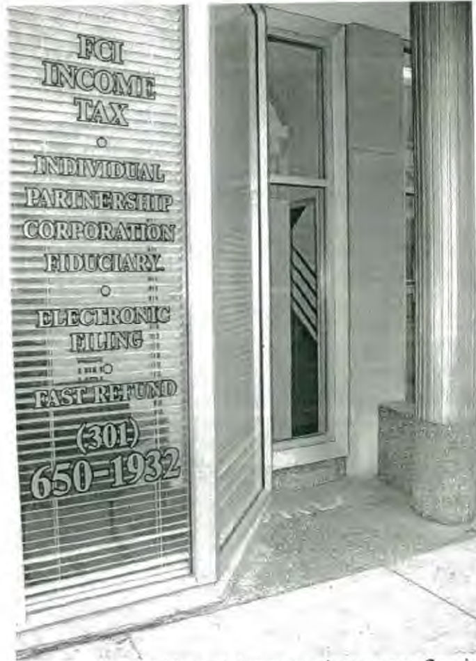
Original aluminum column with partial gray granite terrazzo flooring and newer storefront
