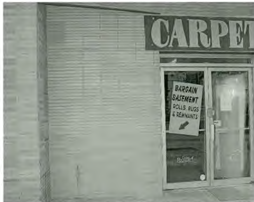
Wall of stretcher course iron-spot brick masonry
