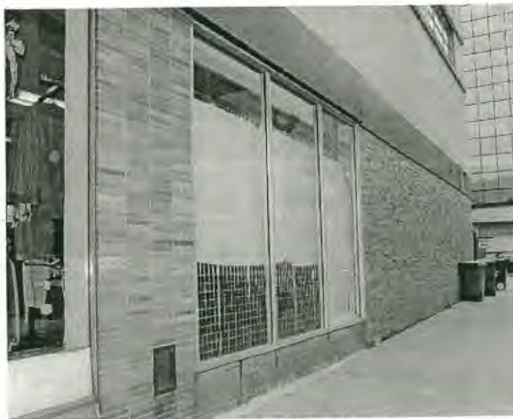
View on Roeder Rd.
