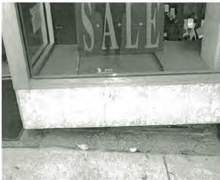
Non-original faux marble kick plate but original gray granite flooring underneath
