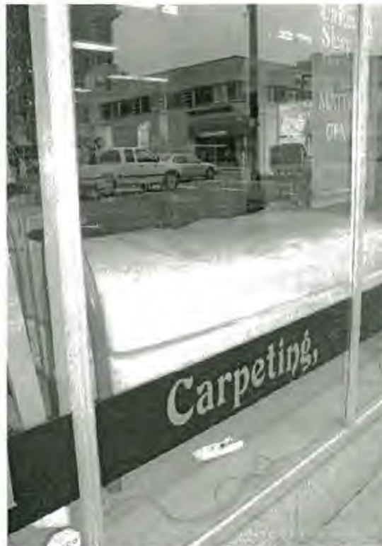
Vertical aluminum storefront window frames
