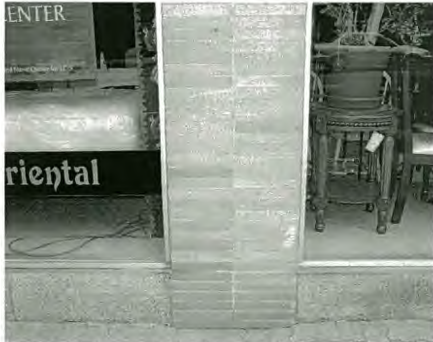
Iron-spot, orange brick laid in all stretcher bond paired columns
