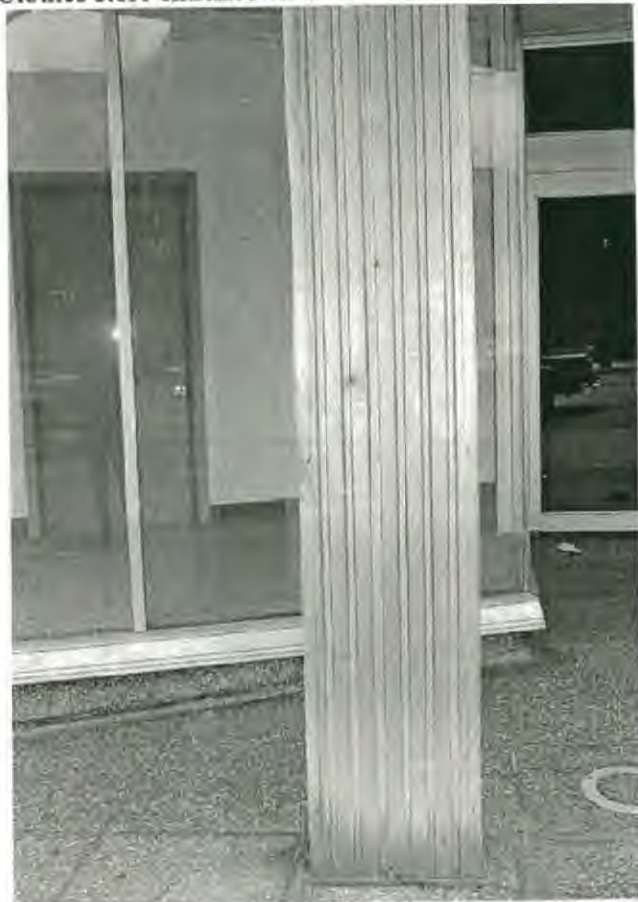
Detail of aluminum encased freestanding column
