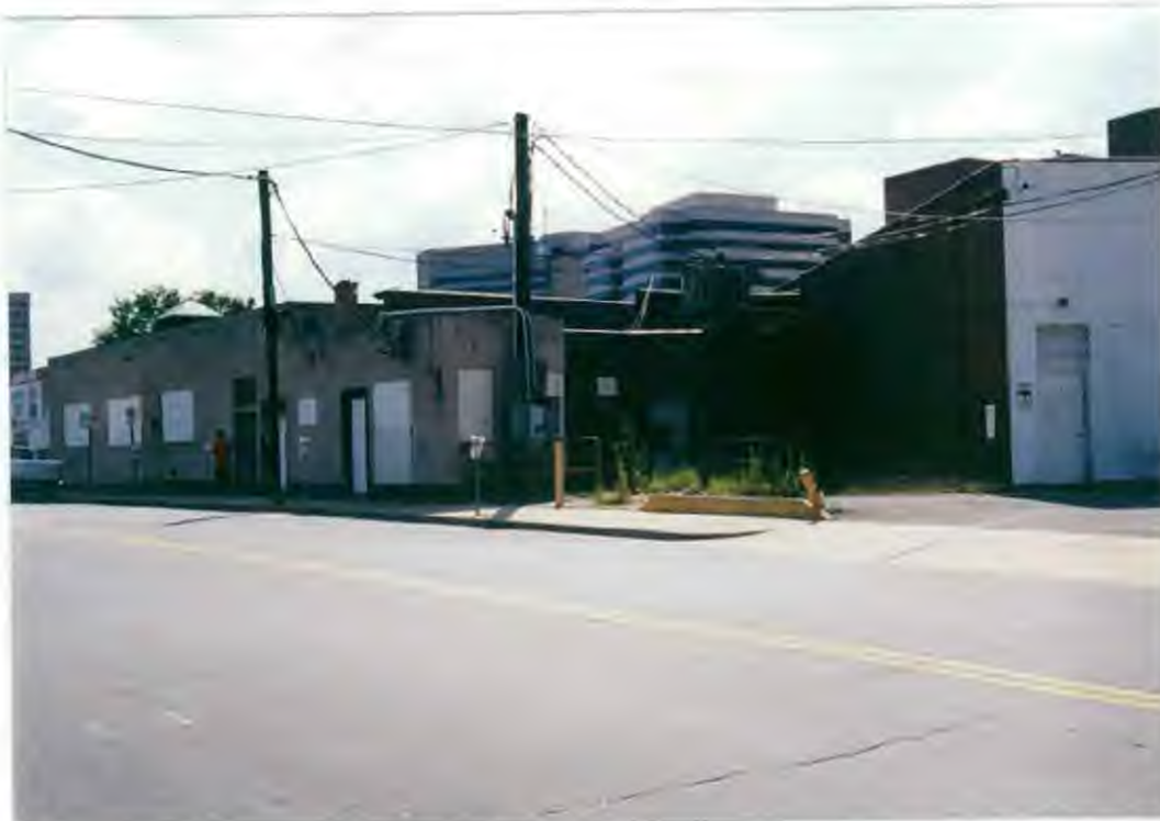
7. REAR OF ELSWORTH DRIVE ELEVATION, SHOWING CURVED END WALL AND SETBACK.
