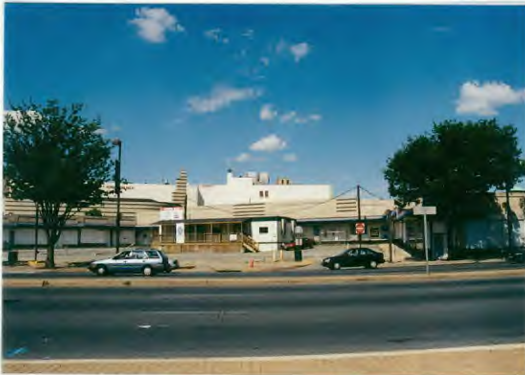
2. OVERALL VIEW OF SILVER SPRING SHOPPING CENTER PARKING COURT.
