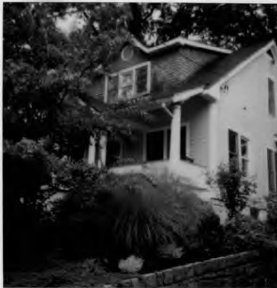
7213 Spruce Ave. T.P. Front/Side
