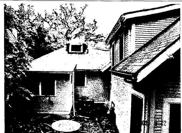
4) Rear patio and West Elevation.
