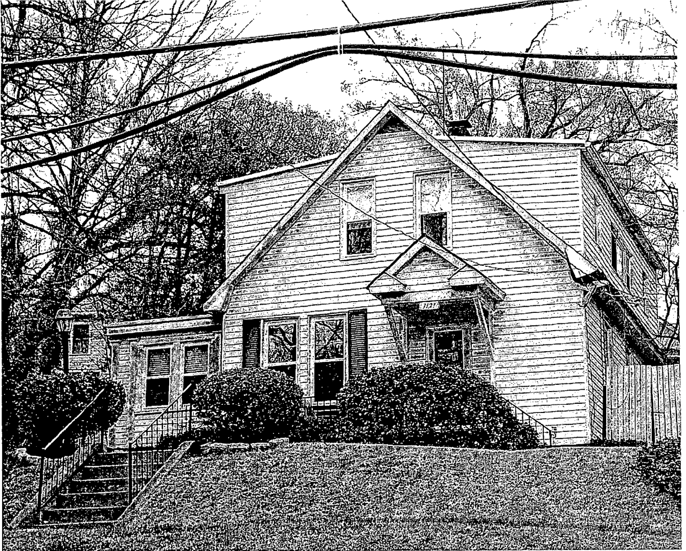
Example of oversized side shed dormers on opposite side of street, same block
