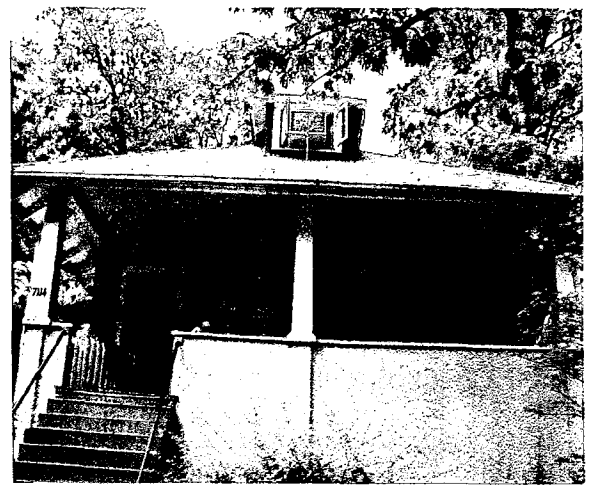
2) East Elevation (facing Poplar Avenue).
