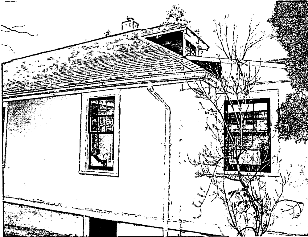
View of north wall of bungalow
