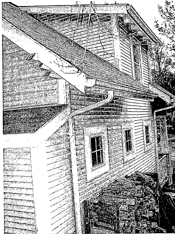
South and west walls of addition
