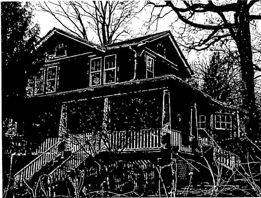
Taller house two up from the subject property to the north
