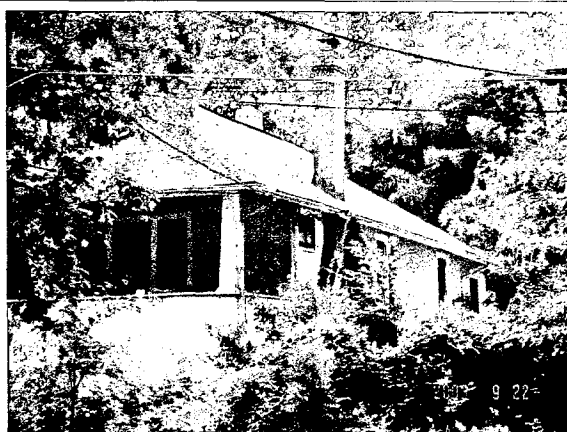
3) View of North Elevation from Poplar Avenue.
