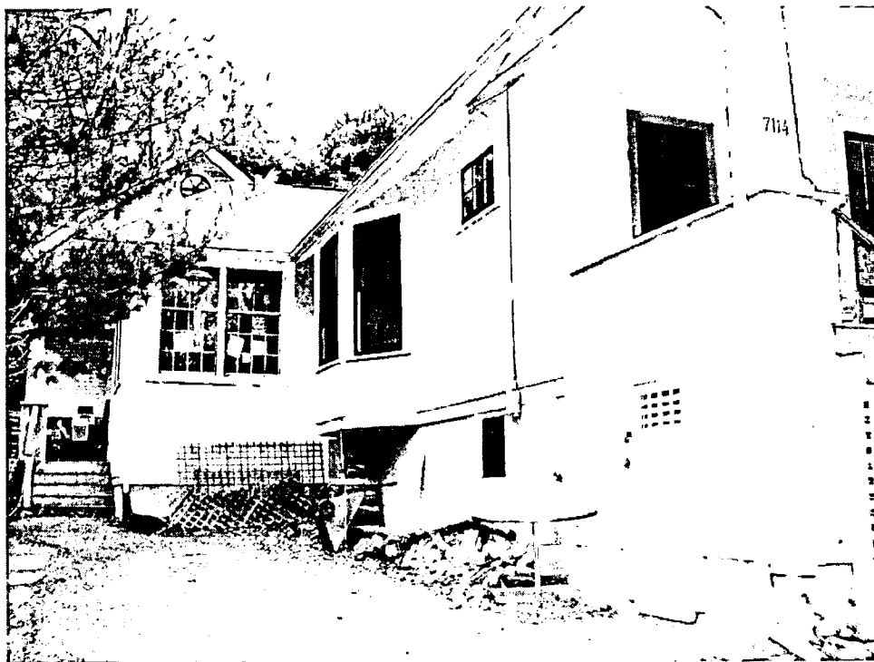
View of south wall of main house with addition at back
