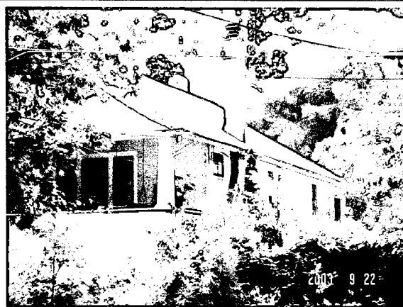
3) View of North Elevation from Poplar Avenue.
