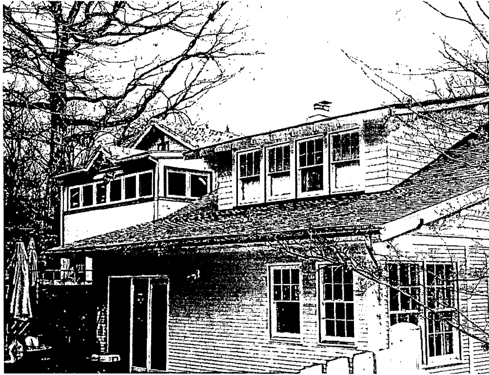
View of original or early shed dormer on rear wall of adjacent yellow house to the north
