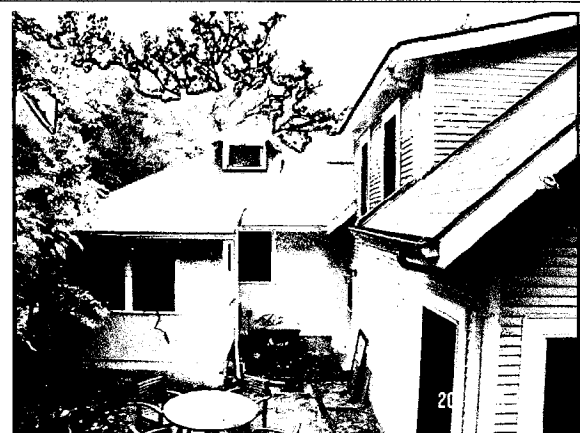
4) Rear patio and West Elevation.
