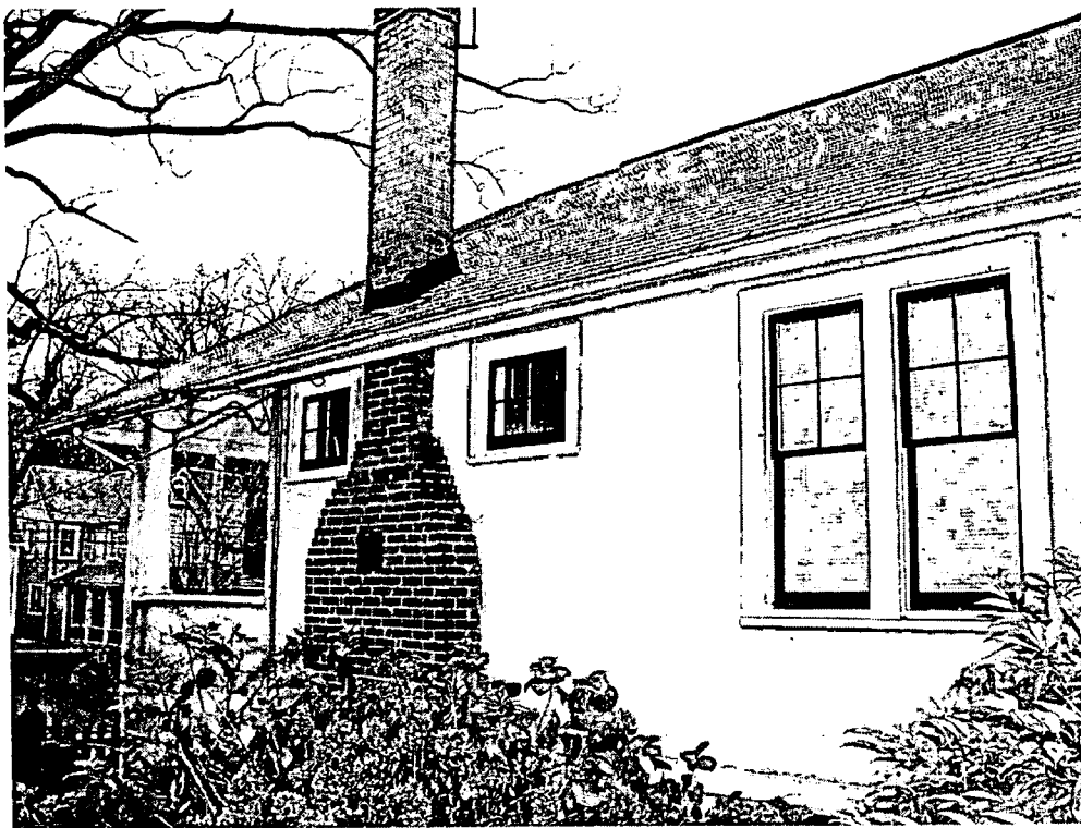
View of front north wall showing brick stack to be potentially heightened
