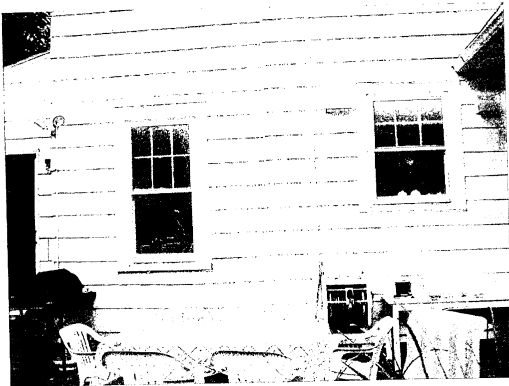
SIDE VIEW (SOUTH)
