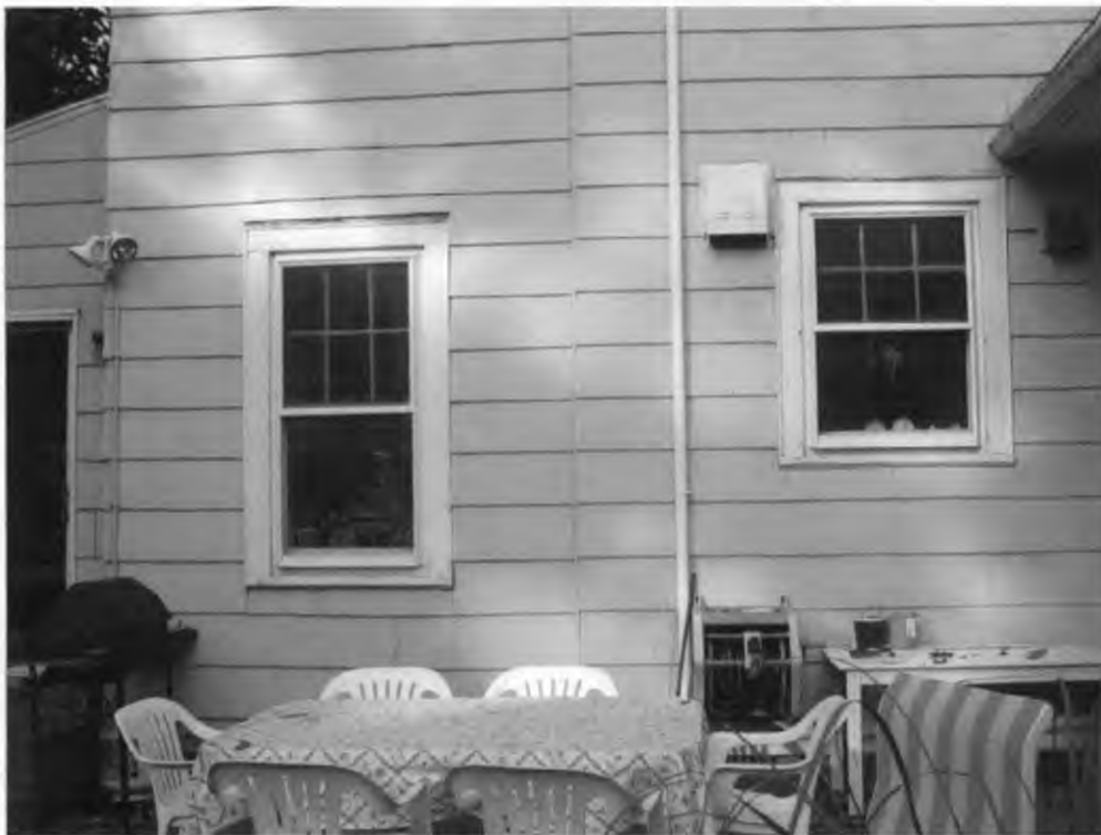
SIDE VIEW (SOUTH)
