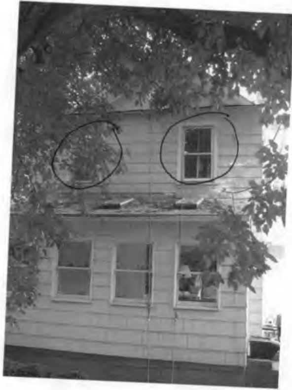
REAR VIEW (WEST)
