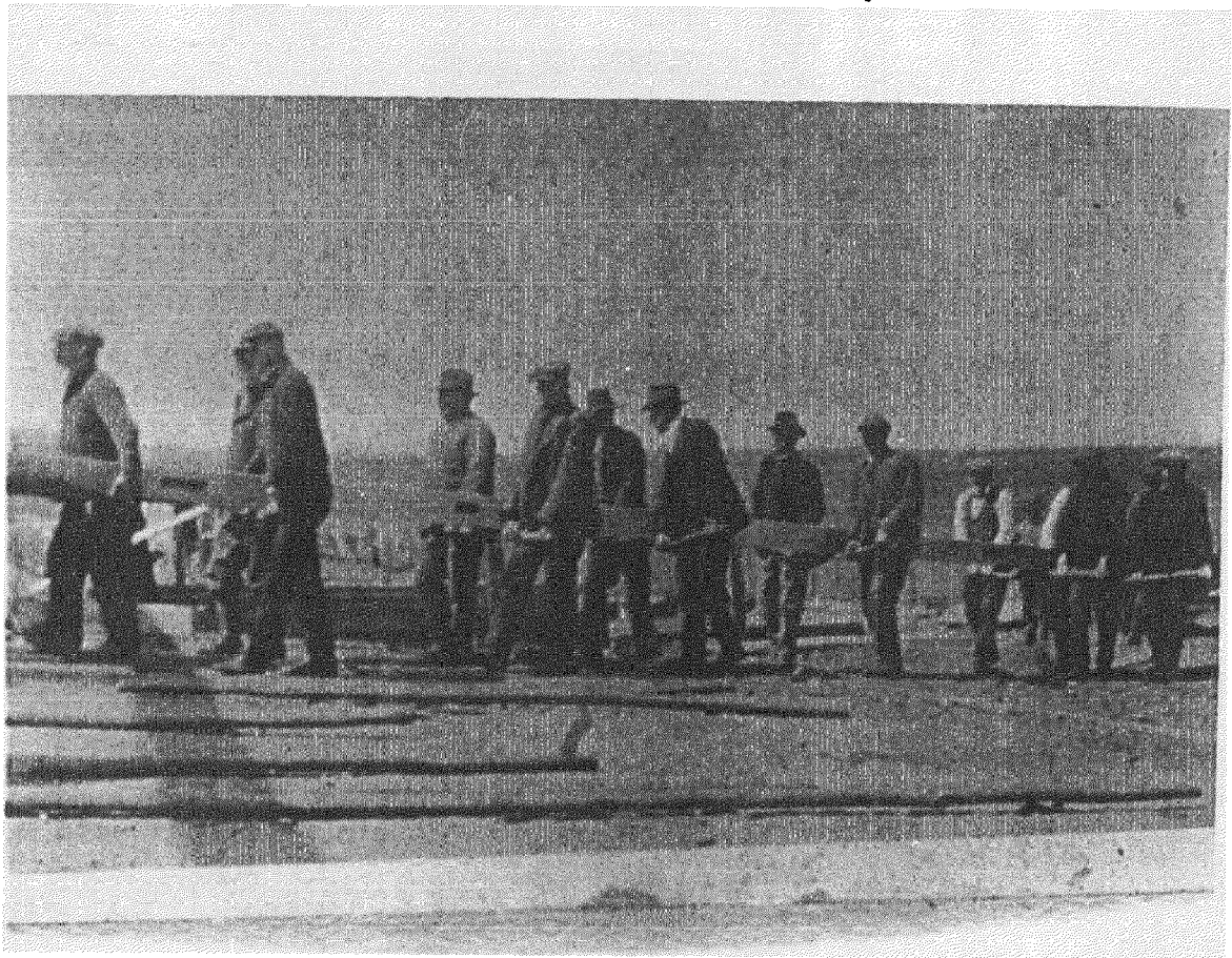
C1985 CONSTRUCTION OF 14-29 BARN (NOW DEMOL'D)
