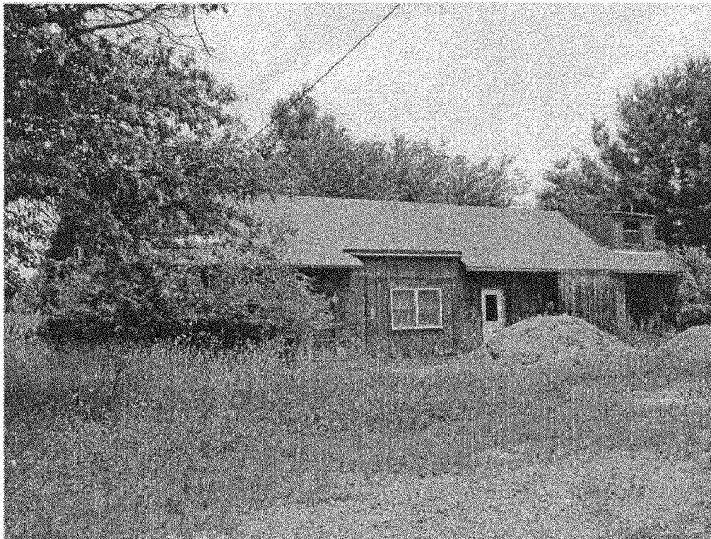
Office (on adjacent parcel P300)
