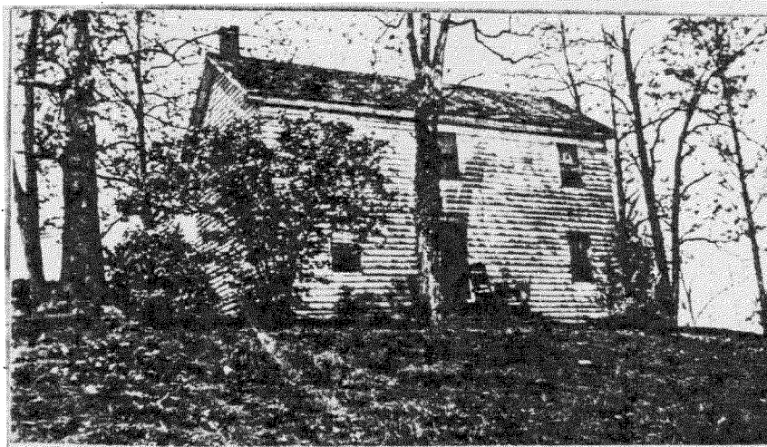
Miller's House at Davis Mill Huntmaster Lane, Germantown Facade: West
