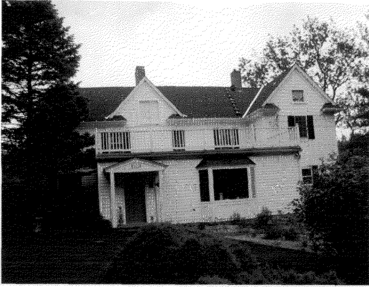
EXISTING REAR SHOWING VINYL SIDING ADDITION
