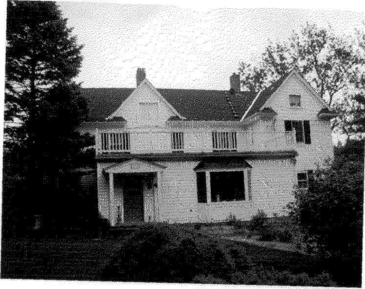
EXISTING REAR SHOWING VINYL SIDING ADDITION
