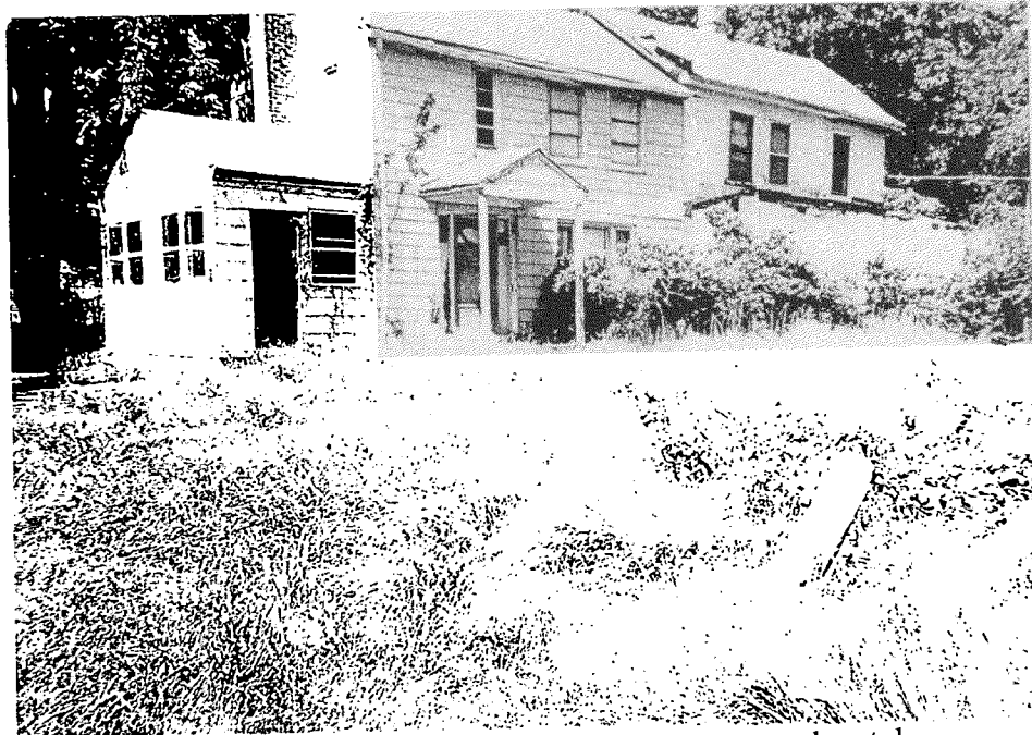
The Boyd House is a 2 story frame house of a vernacular style probably typical of Maryland farm houses at the turn of the century.
