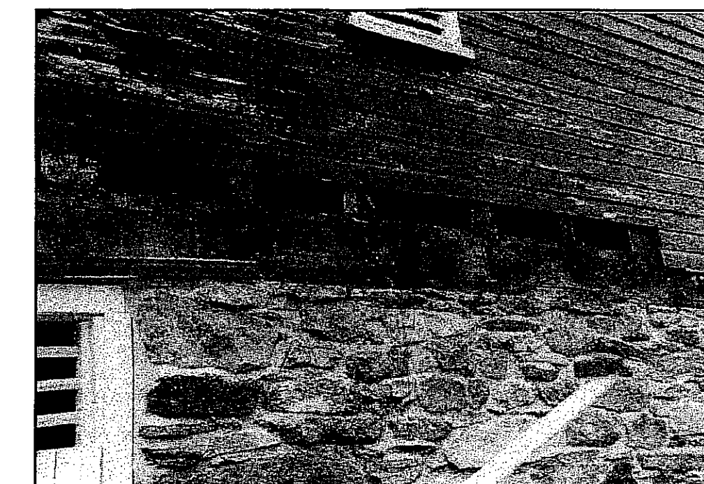
PHOTO #8 - EAST ELEVATION
