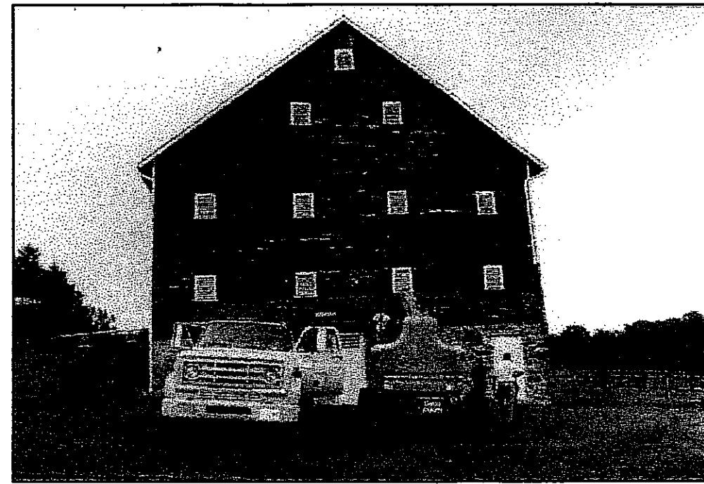
PHOTO #1 - EAST ELEVATION
