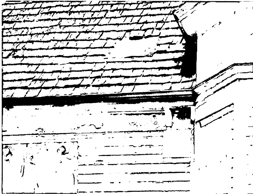
Roof and wall patches.
