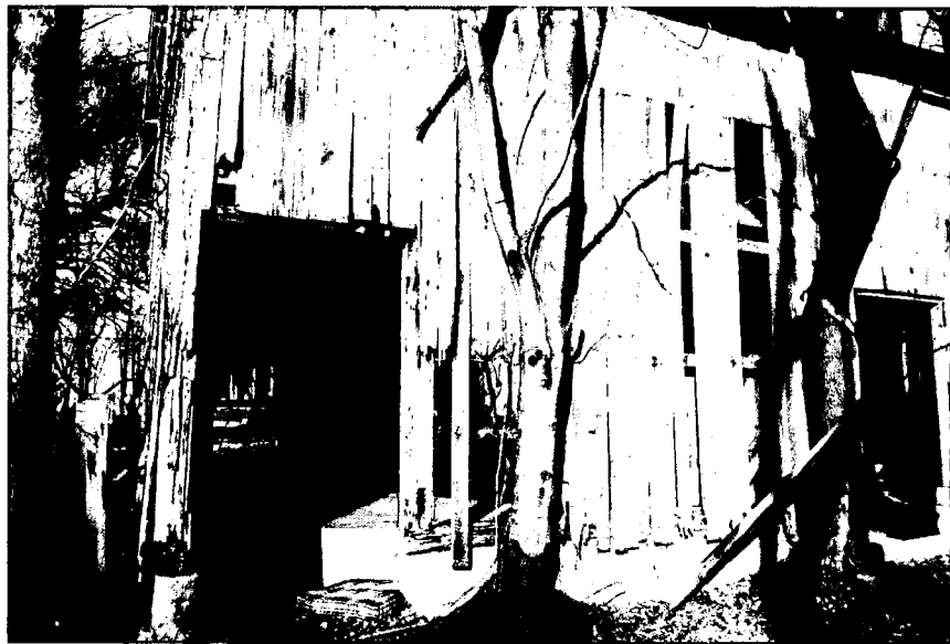
Deteriorated & missing barn siding before emergency stabilization
