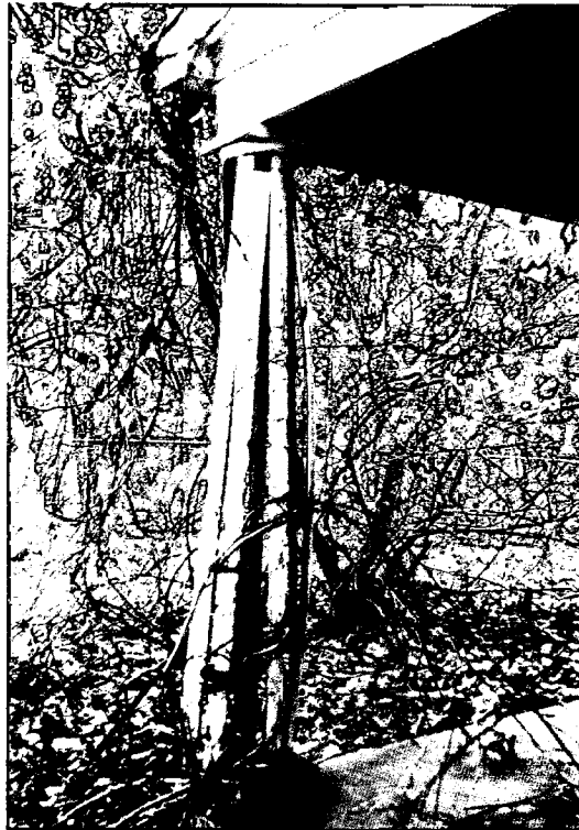
Collapsing column at east porch
