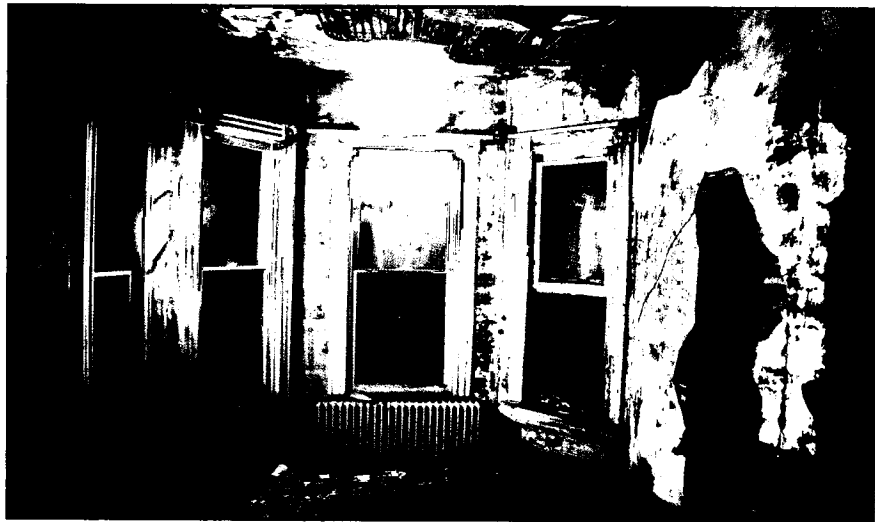
Windows in Stair hall
