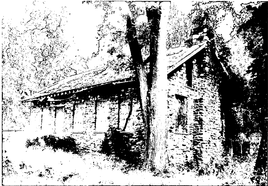
Stone House view from Southwest before emergency stabilization
