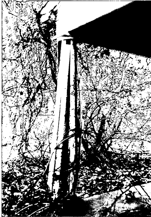
Collapsing column at east porch
