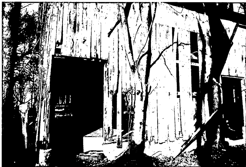
Deteriorated & missing barn siding before emergency stabilization
