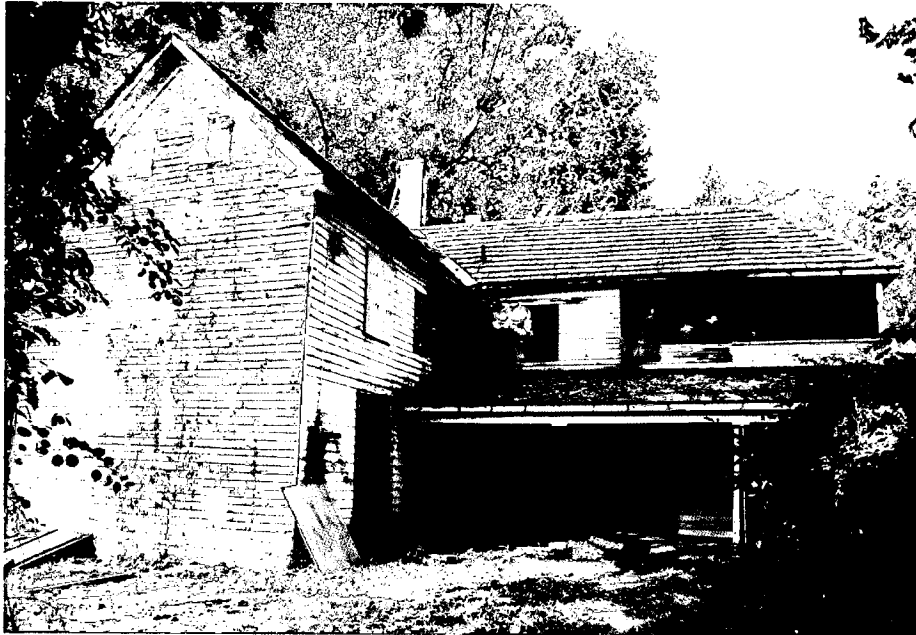
Main House view from Northeast – Before emergency stabilization
