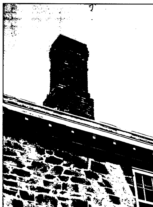
Detail Southwest Chimney
