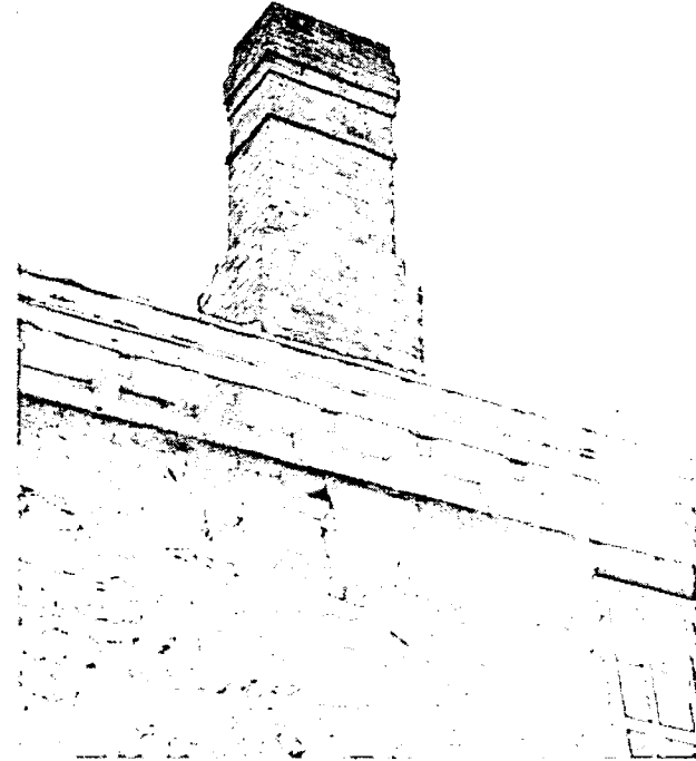
Detail Southwest Chimney
