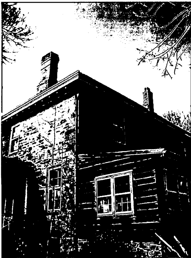
Northeast Elevation - Detail
