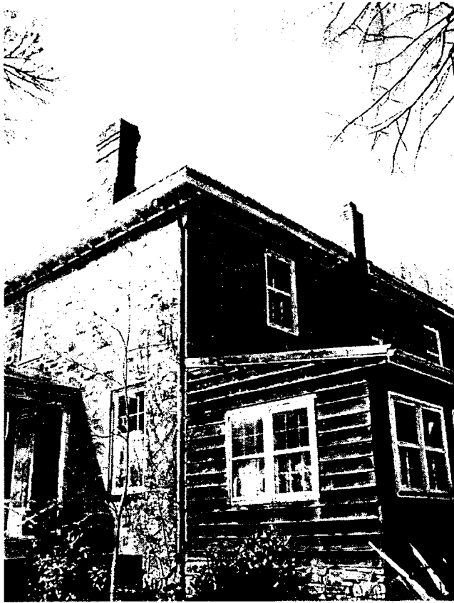
Northeast Elevation - Detail
