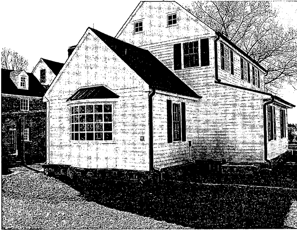
Site of areaway stairs
